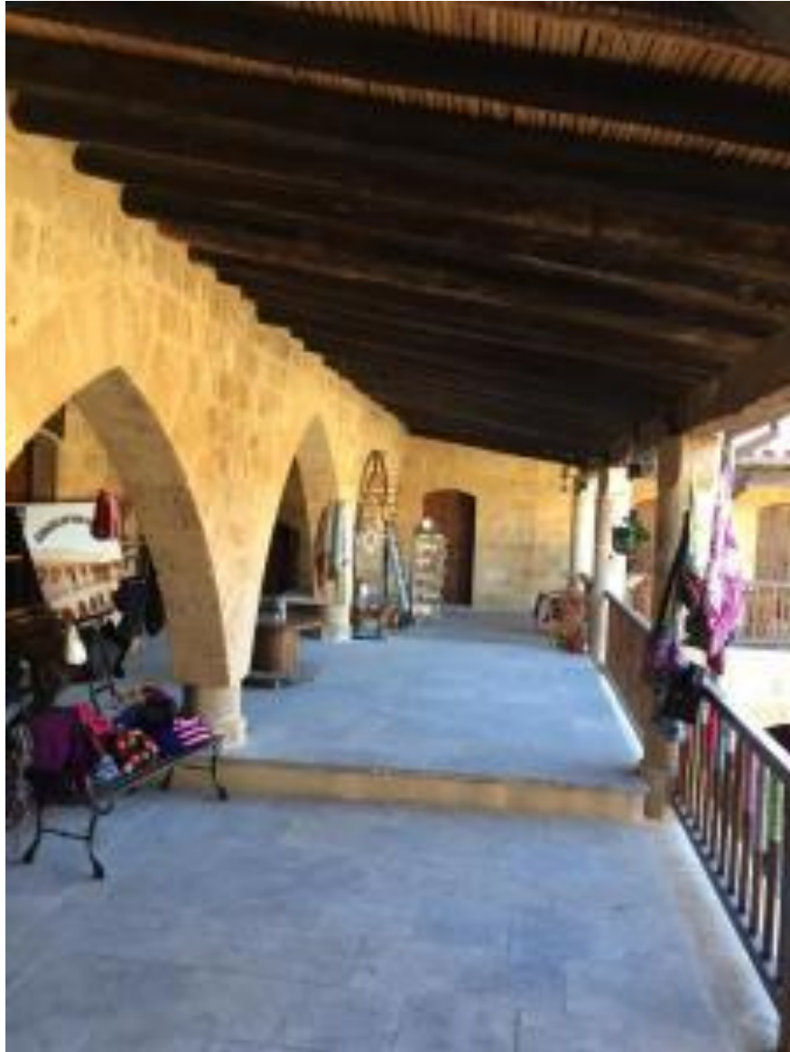
Figure 3.44: Conserved structure in Kumarcılar Hanı . (Author, 2017)
