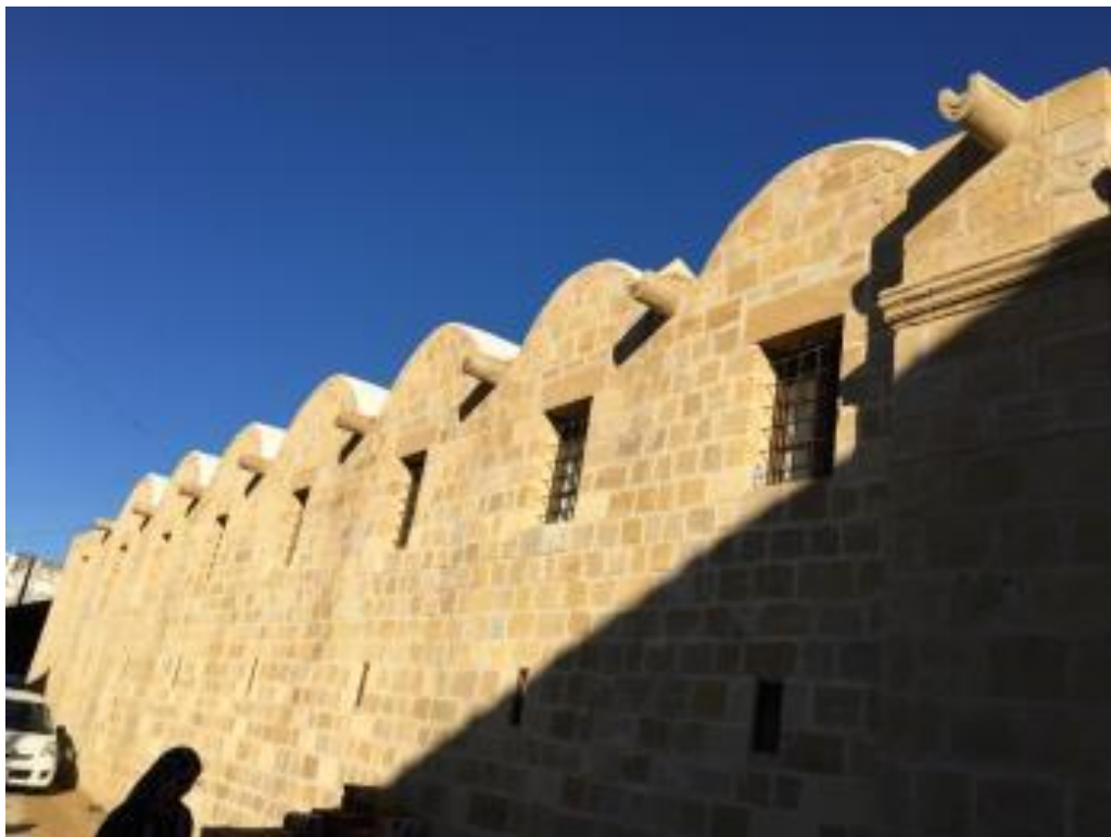
Figure 3.42: Conserving architectural elements in Kumarcılar Hanı. (Author, 2017)
