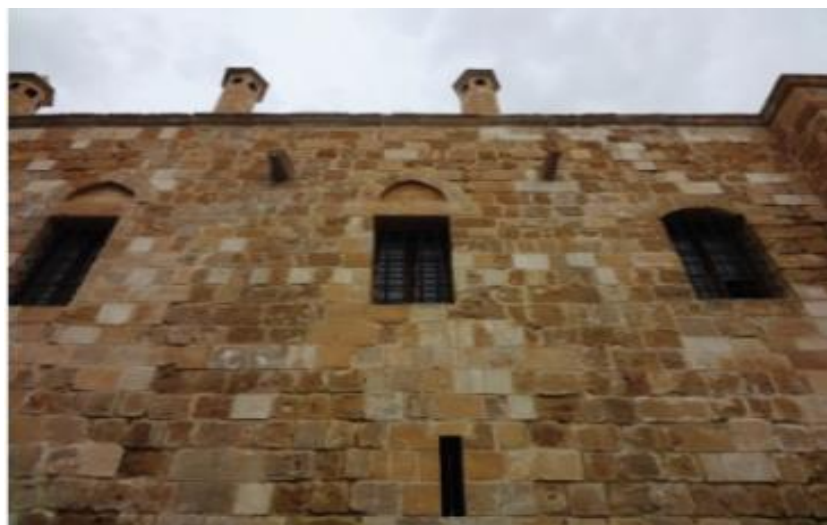
Figure 3.22: Büyük Han-North Elevation showing octagonal chimneys on the roof of the building. (Author, 2017)
