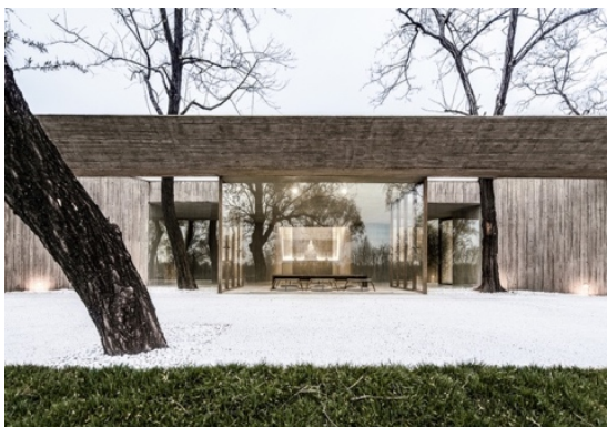
Figure 53: Courtyard View (URL 26)
