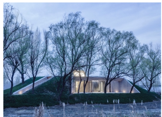
Figure 54: Courtyard View (URL 21)
