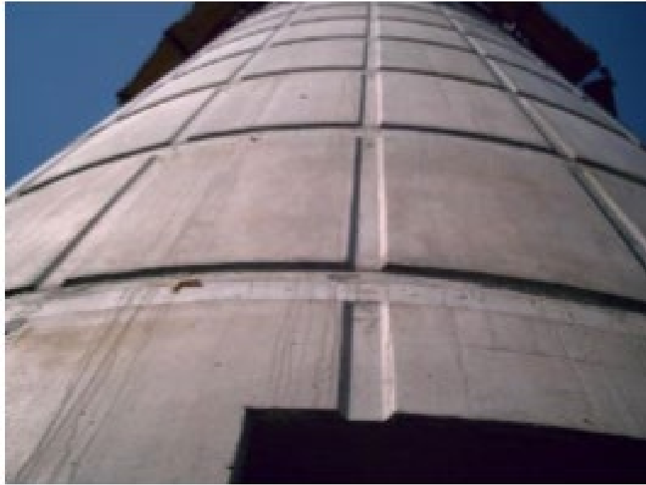
Figure 2: Good surface finish by using SCC without any repairs, Perham tower
