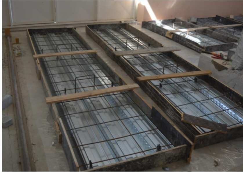
Figure 3.8: m-k test specimens before concreting.
