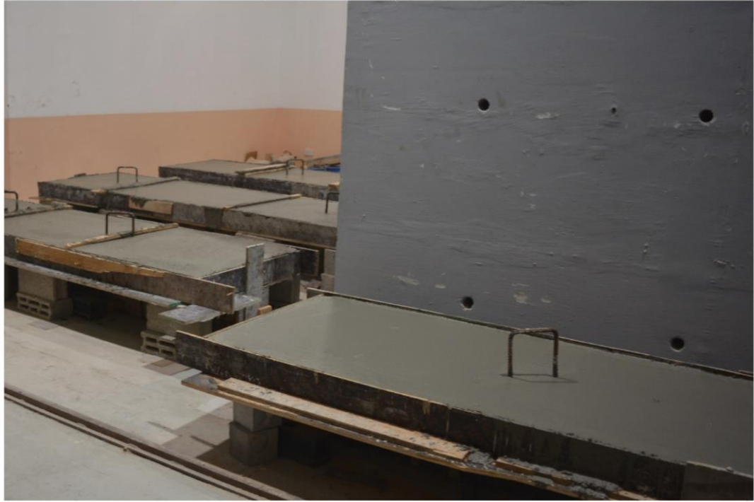
Figure 3.4: Static test specimens after concreting.
