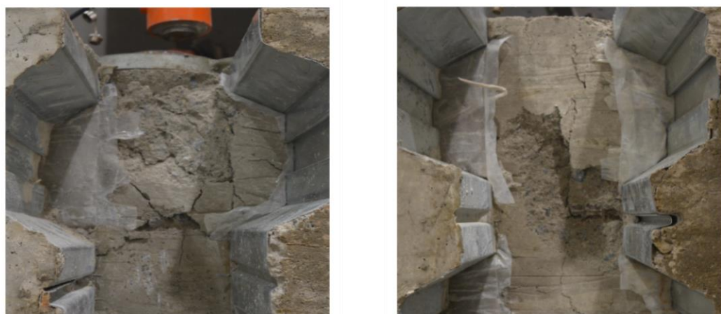
Figure 4.26: Failure mode of specimen series SC-FR with local crushing of the beam.
