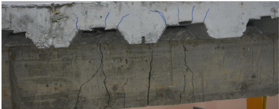
Figure 4.5: CS-SC2 specimen beam and slab cracks after failure.
