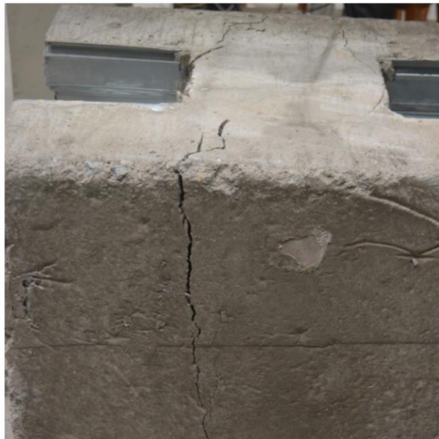
Figure 4.34: Mode of failure for specimen series of SC.
