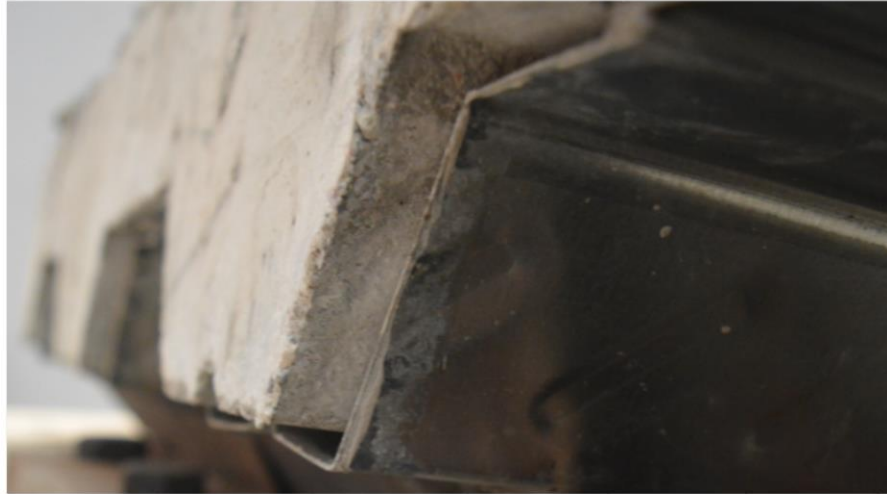
Figure 4.14: End-slip of specimen mk-SS1s after failure.
