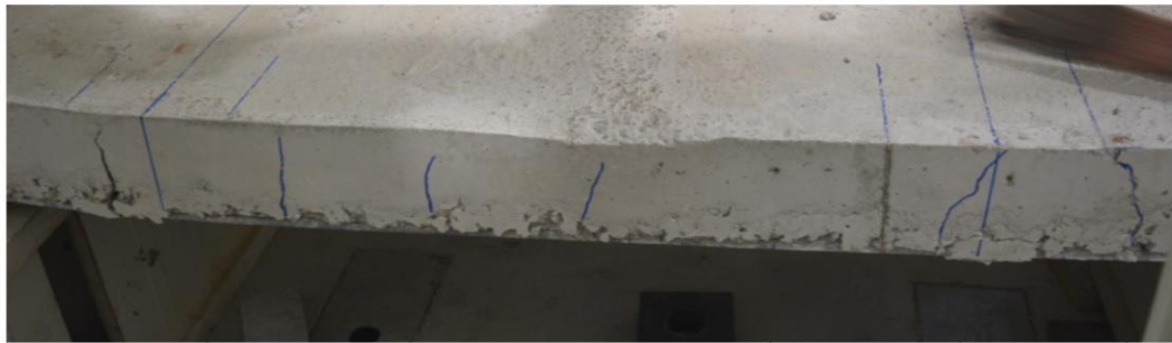
Figure 4.15: Overall view of mk-SS1s specimen after failure due to the failure at the location of the left line load.
