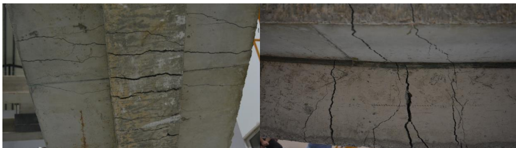
Figure 4.7: The failure modes of the SS sample.
