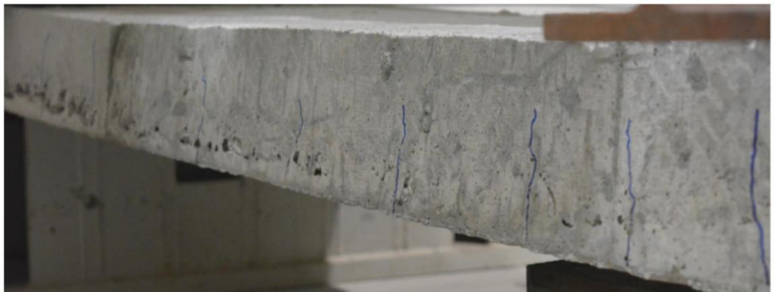
Figure 4.19: Pattern of cracks after failure for specimen mk-LS1s.
