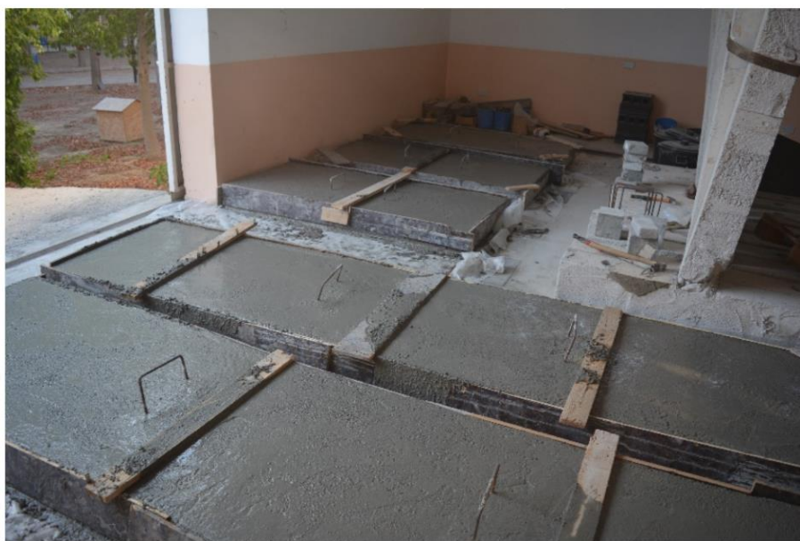
Figure 3.9: m-k test specimens after concreting.
