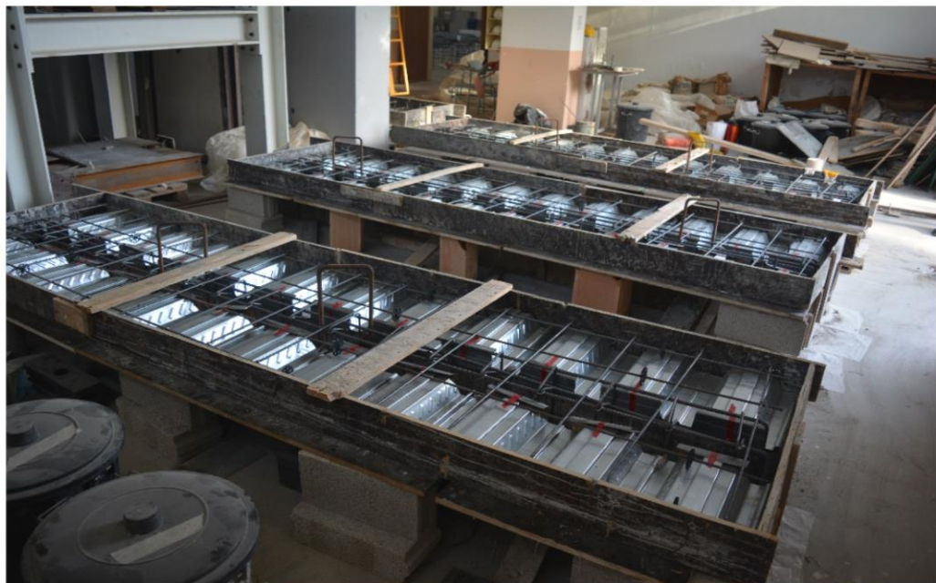
Figure 3.3: Static test specimens before concreting.
