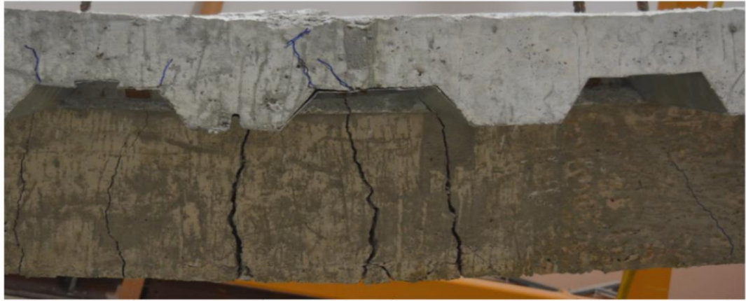
Figure 4.4: CS-SC1 specimen beam and slab cracks after failure.
