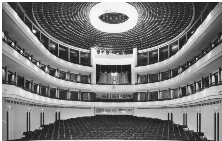
Figure 21: Main auditorium of Vahdat Hall located in Tehran, Iran URL-10
