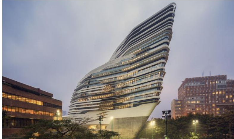
Figure 19: The Jockey Club Innovation Tower by Zaha Hadid (Kothawade, 2017).
