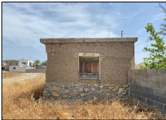
Figure 8: Example of the single unit/units without hall in Mesarya Region (Author, 2019)
