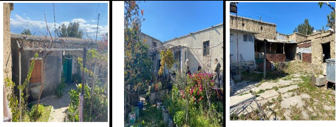
General views of the dwelling interior
