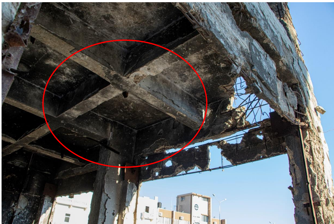
Figure 4.4: The Elastic Deformation in The Beam
