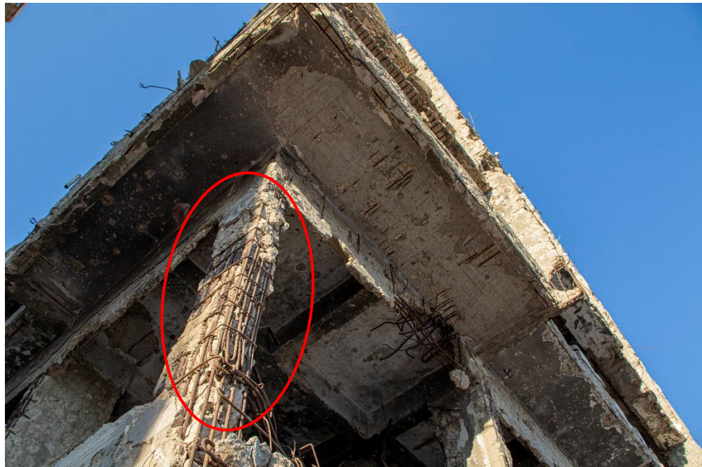
Figure 4.6: Good Steel Reinforcement Bonding
