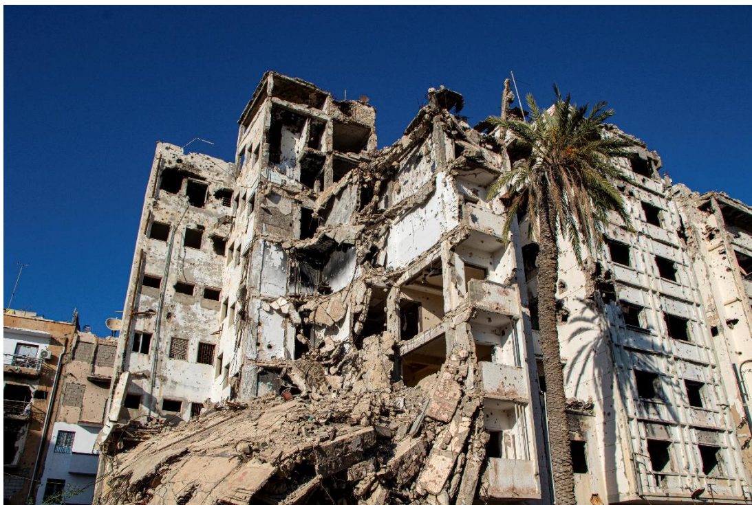
Figure 4.9: Partial Collapse
