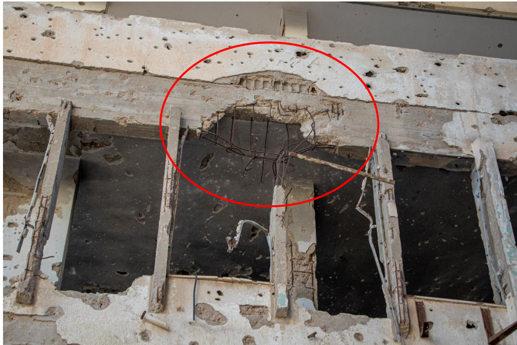
Figure 4.8: Fragmentation and Loss of Materials
