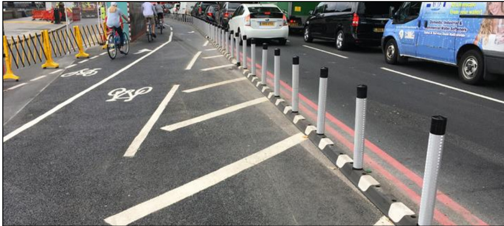
Figure 50: Narrow Cycle Defender Incorporating Wands (Rediweld, 2020)
