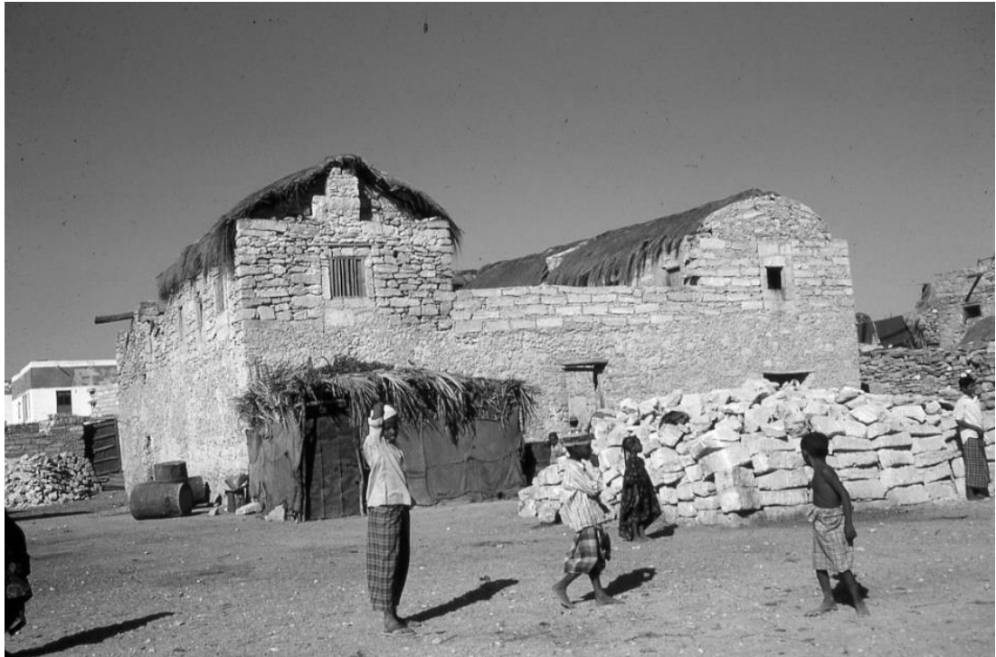
Figure 15: Traditional House in Taqa, Dhofar. By Development Workshop Digital Archive, licensed under CC BY-NC 4.0
