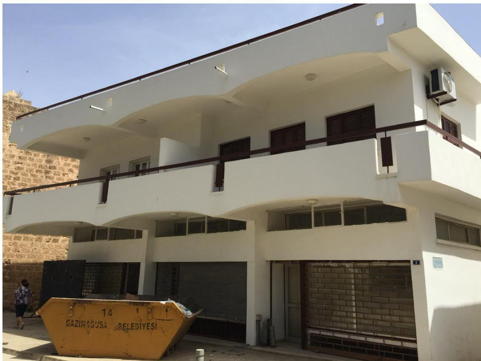
Figure 34: Approach view of Efecan Building Complex; (Author, 2019)
