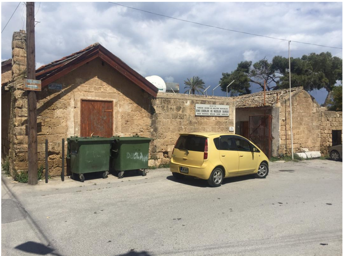
Figure 42: The approach view of the Old Police Station; (Author, 2019)
