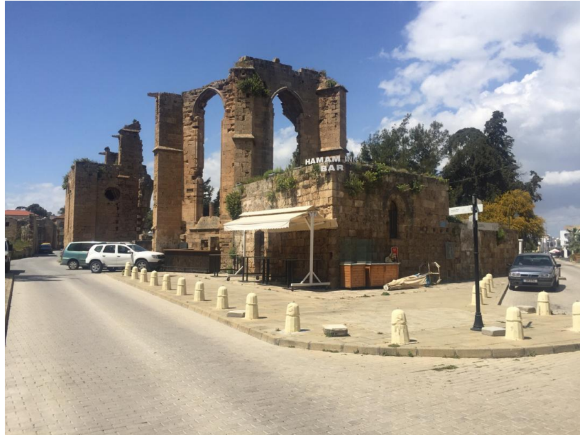
Figure 21: The approach view of the Cafer Pasha Hammam ; (Author, 2019)
