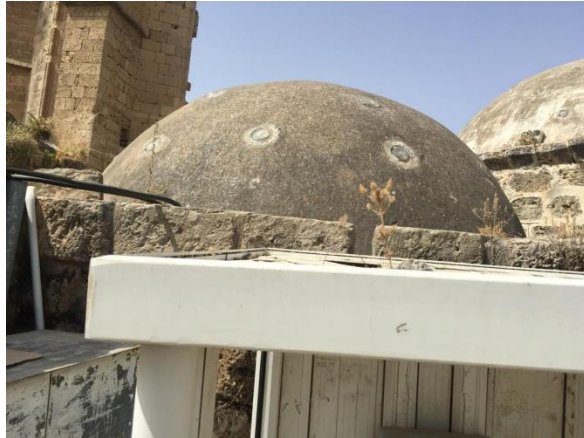
Figure 19: The dome of the Hammam and opening the dome. (Author, 2019)
