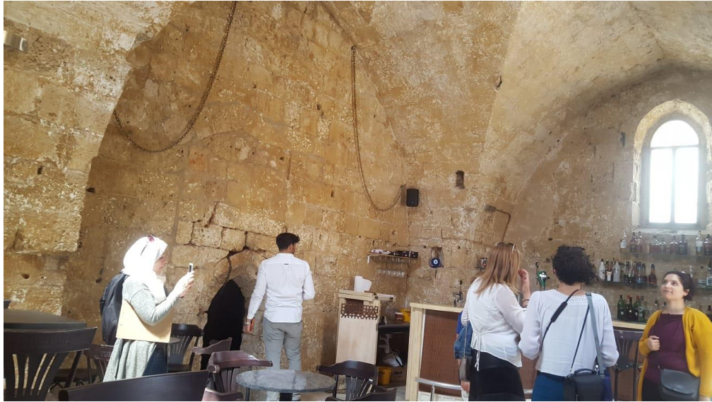
Figure 22: Interior of the Cafer Pasha Hammam; (Author, 2019)
