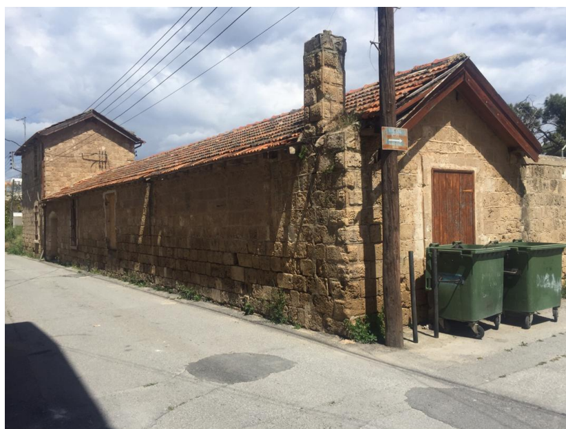
Figure 41: The exterior view of the Old Police Station; (Author, 2019)
