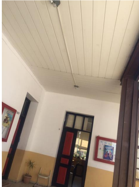
Figure 24: The ceiling and steel column; (Author, 2019)
