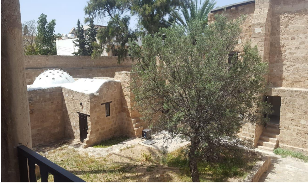
Figure 9: The female part of the Chimney House with its courtyard and also showing the small Hammam (bathhouse); (Author, 2018)
