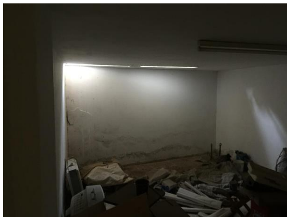
Figure 36: Showing basement of Efecan Building Complex; (Author, 2019)
