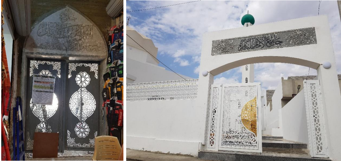
Figure 65: Rebuilding the Mosques in the old city of Mosul valuing the original elements
