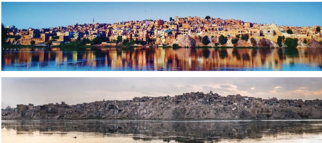
Figure 56: The panorama of the old city of Mosul before and after the war. The credit of the upper image to Mosul municipality and the lower image has been taken by Musaab Sami Al-Obeidy
