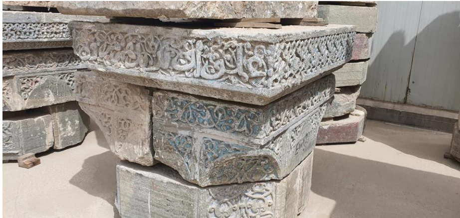
Figure 62: The preserved and secured original material They will be a base for Al Nuri Mosque and Hadbaa Minaret reconstruction process Source: Bashar Al Talib
