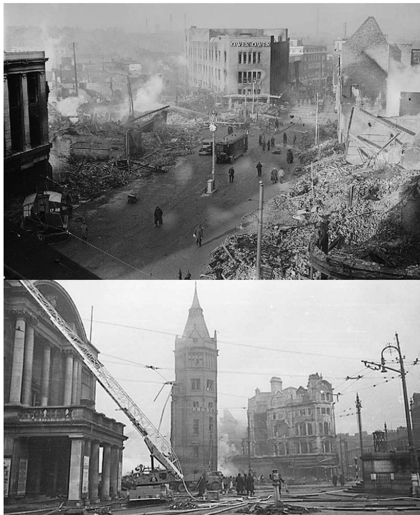
Figure 10: Damaged pictures of Coventry City
