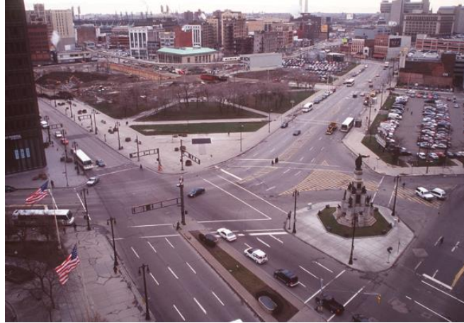
Figure 19: Dupont Circle Before Renovation. (Retrieved from https://www.craigslist.com/membership )
