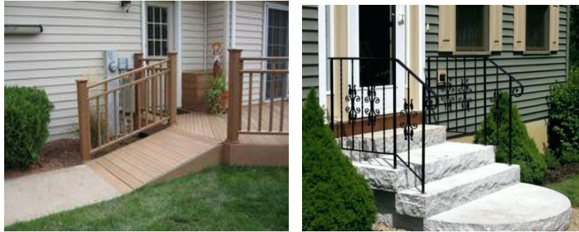
Figure 23: Handrails and Ramps for Entrances (URL 17)
