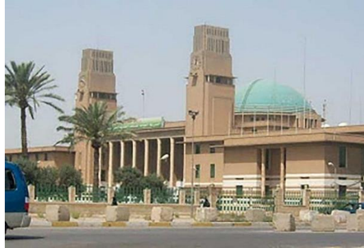
Figure 45: Buildings from Iraqi Architecture (URL38)
