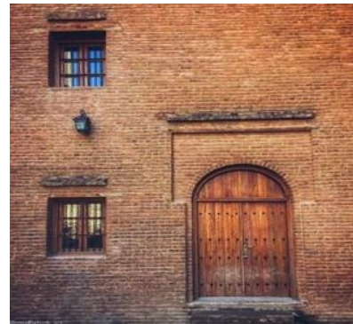
Figure 63: Enclosed Façade from Outside (Author)
