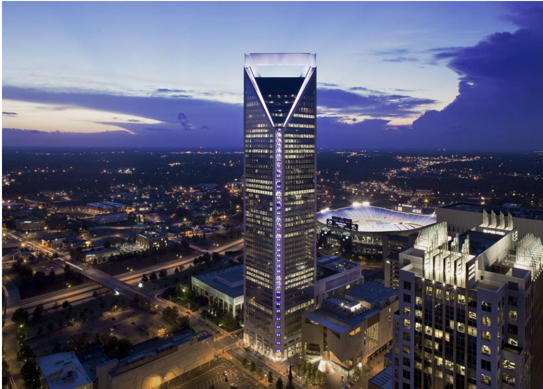
Figure 4.7: Duke Energy Center Interactive Facade with 45,000 LED Lights (S & ME, 2020)
