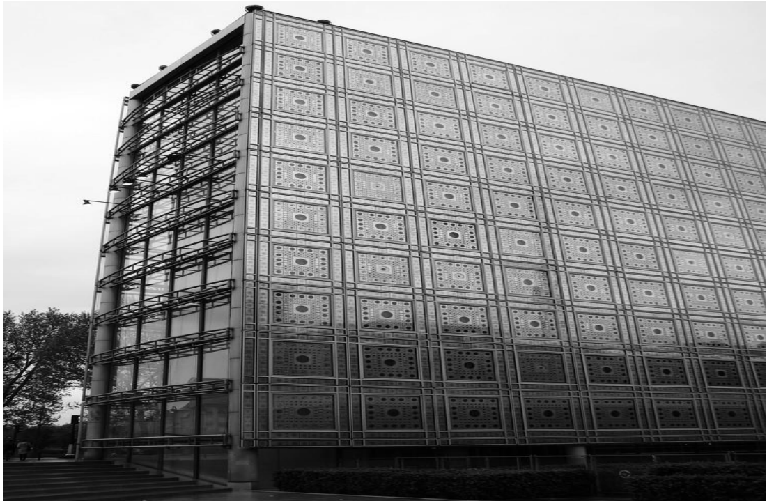
Figure 4.9: The Southern Façade of the Arab World Institute (Winstanley, 2011)
