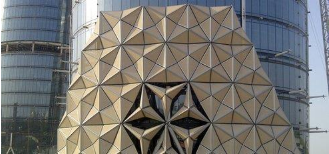
Figure 2.13: Al Bahar Tower's Adaptive Facade in form of Curtain Wall (Cilento, 2012)
