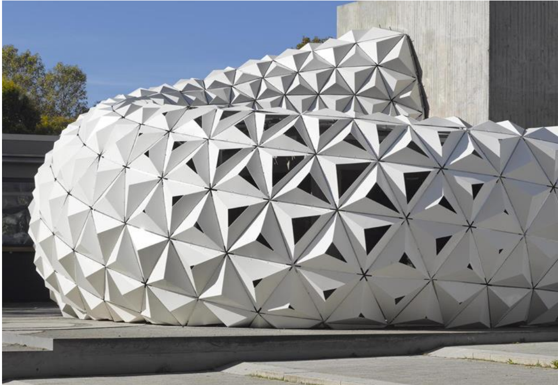
Figure 3.9: A pavilion Made of Bioplastic in Stuttgart (Griffiths, 2013)
