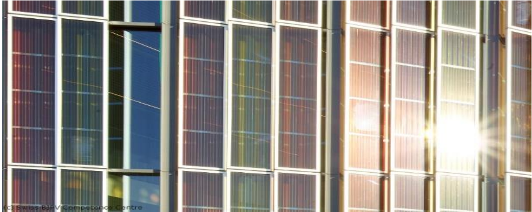
Figure 3.10: SwissTech Convention Center Facade with PV Panels Embedded in Glassy Structure (BIPV, 2019)
