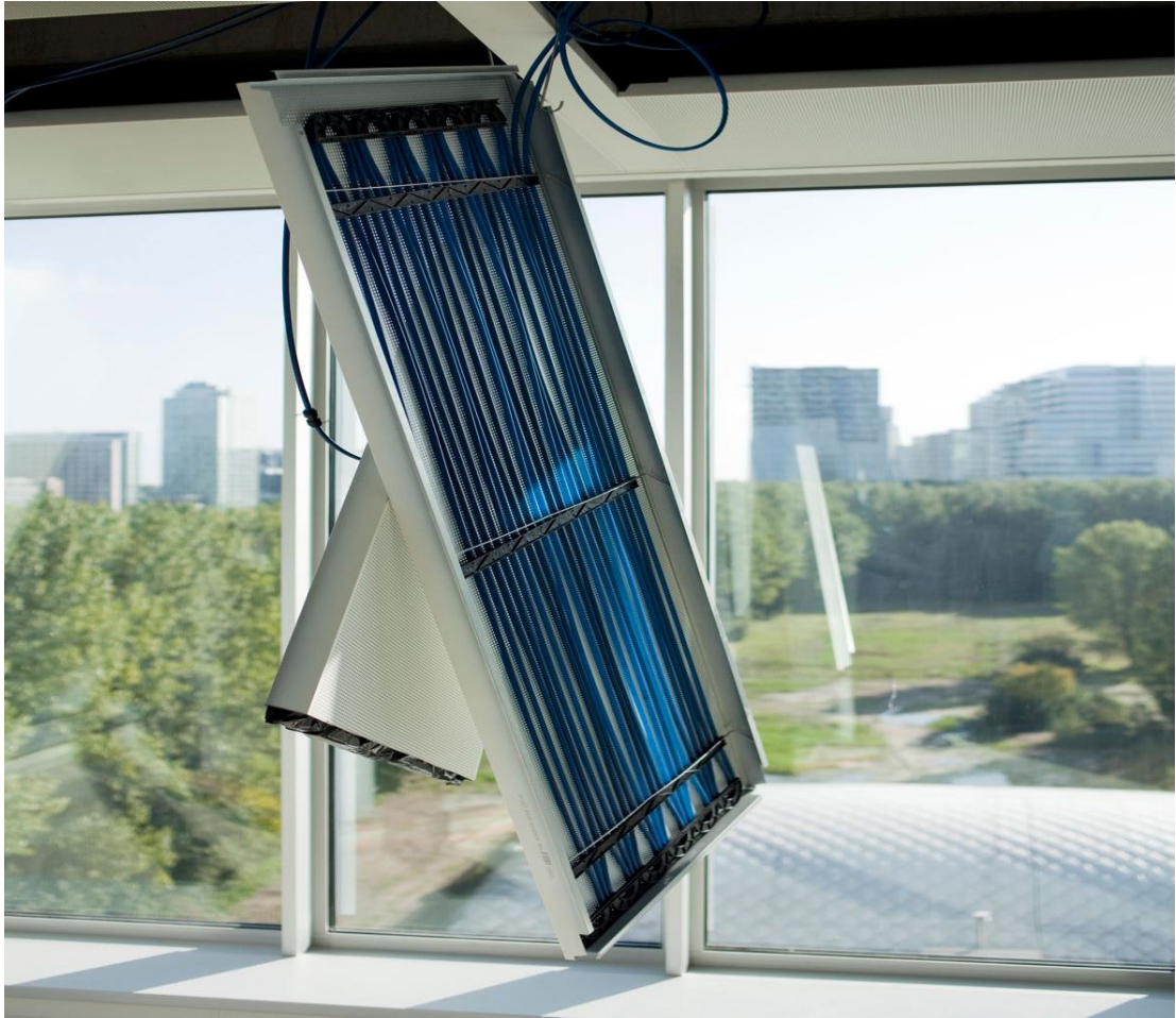
Figure 2.5: The LED Lights Powered by Ethernet Cables (Bloomberg, 2015)
