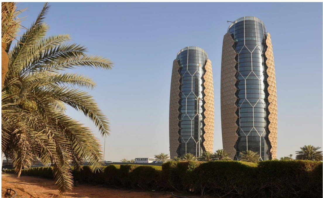
Figure 4.15: The Facade of Al Bahr Towers Consists of a Curtain Wall (Cilento, 2012)
