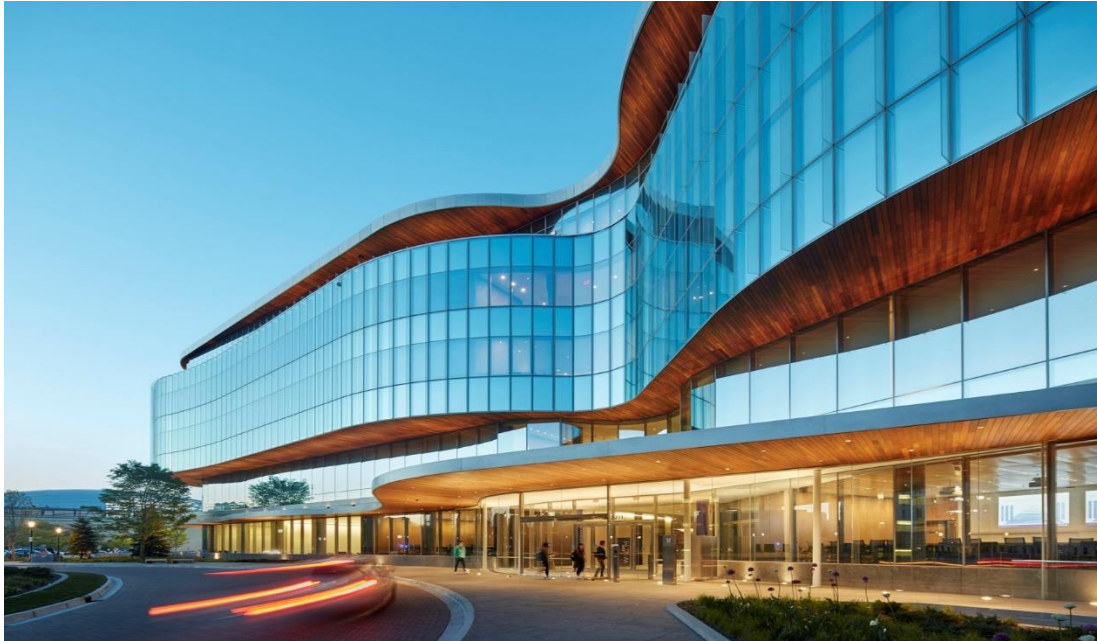
Figure 3.8: Kellogg School of Management Glasses are Enhanced with Aerogel Panels (Gonzalez, 2018)
