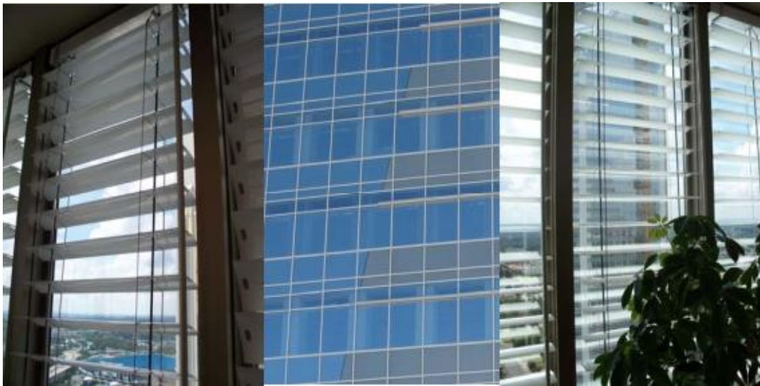
Figure 4.8: Duke Energy Center Daylight Harvesting Blinds (Duke Energy Center, 2020)
