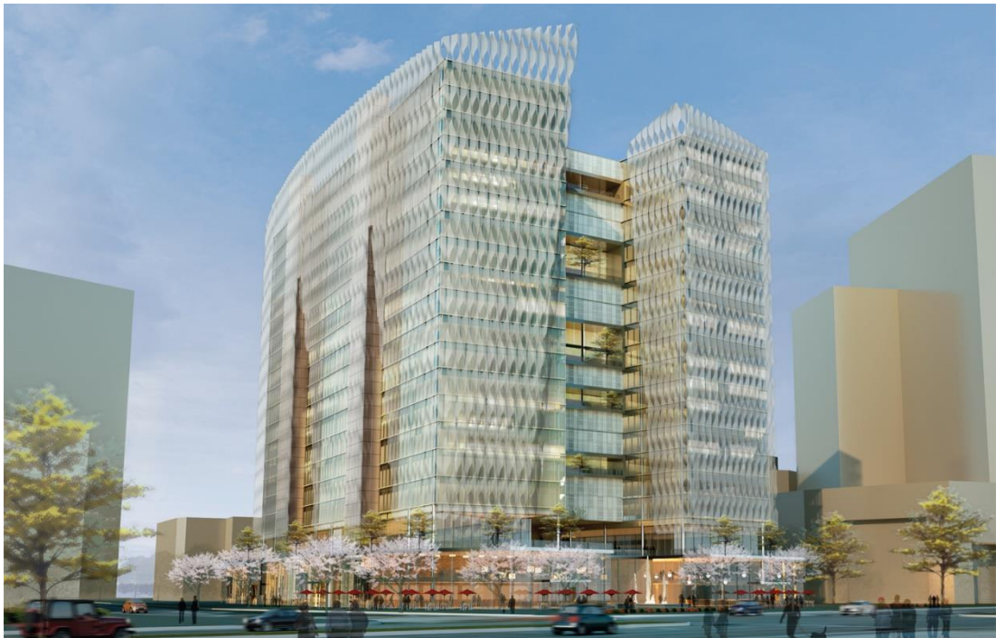
Figure 3.13: Dynamic Shading Layers Made from EAP (Architizer, 2019)
