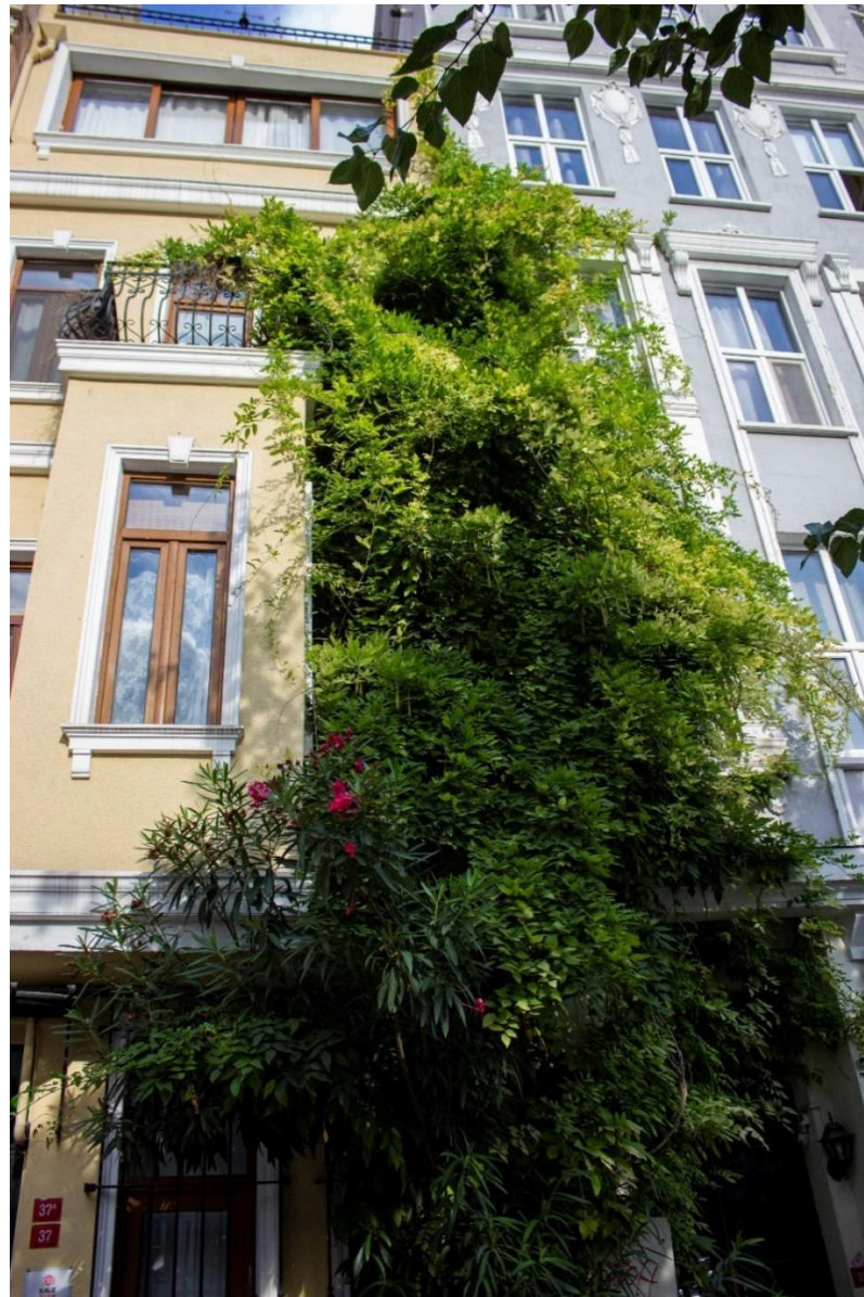
Figure 3: Vertical green system, Direct Climbing Green Facade on residential buildings in Istanbul, Turkey (by Author).
