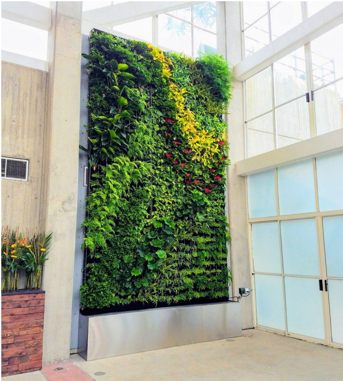
Figure 6: Vertical green system, hydroponic living wall ("San Francisco Zoo vertical garden", 2021).
