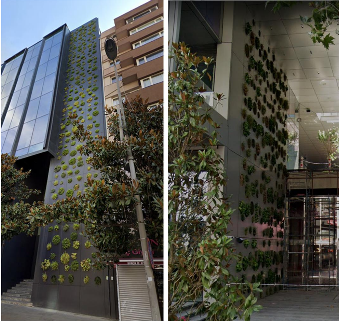
Figure 8: Vertical green system, vertical substrate-based living wall, integrated modules, Garanti BBVA in Istanbul, Turkey (by Author).
