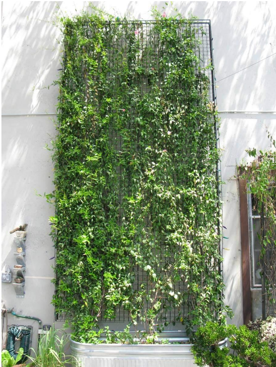
Figure 4: Indirect Climbing Green Facade (Green Wall SG).
