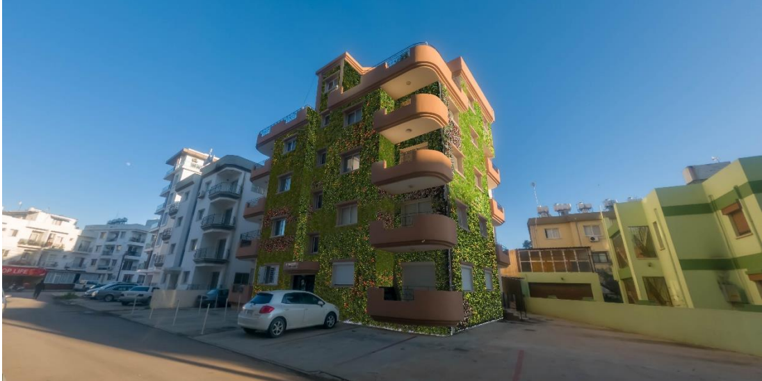
Figure 39: Döveç Apartment 20 in Karakol district after green surface system integration (by Author).
