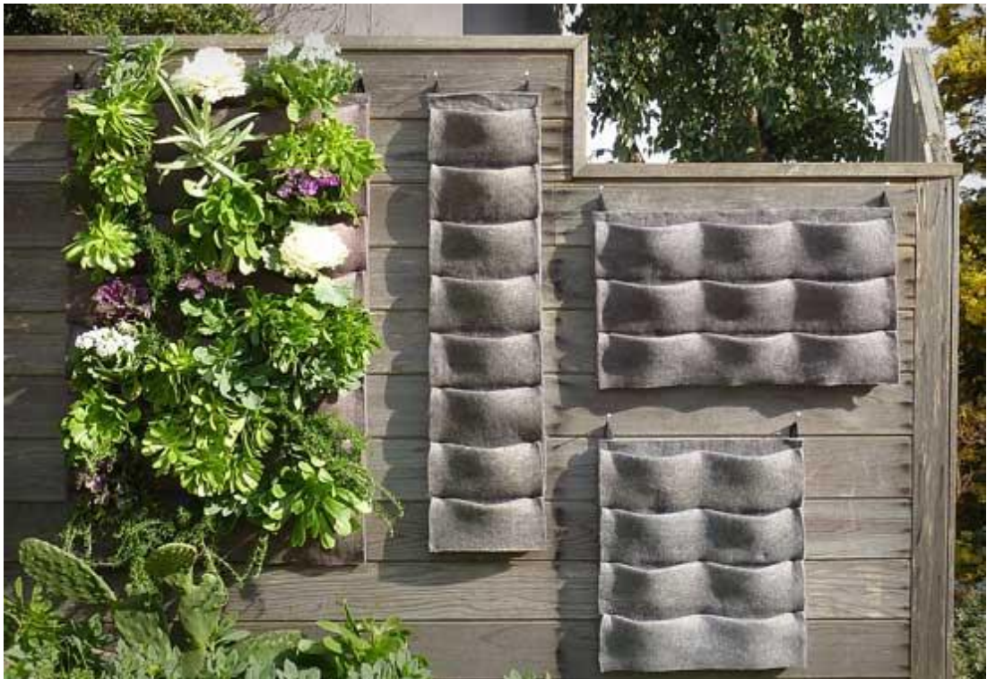
Figure 18: Modular flexible bags living wall (Tarboush, 2019).
