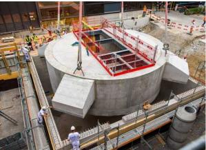
Figure 6: The concrete cylinder that encloses the centrifuge was already placed in August 2020.
