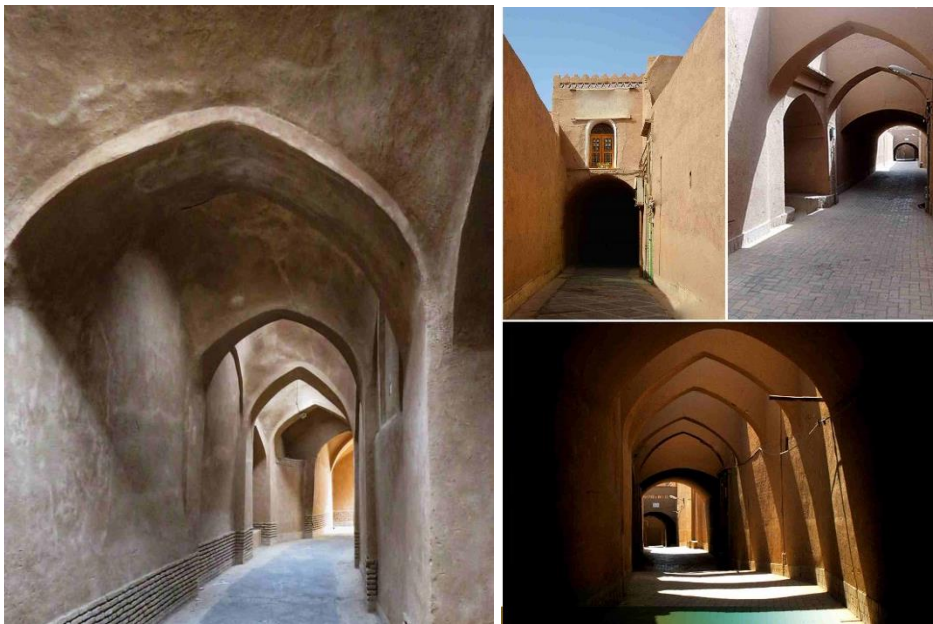
Figure.5.4. Earth Architecture and Sabat Structures (URL 29)
