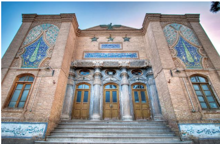
Figure.3.25. Main Entrance of Markar School (URL 10)
