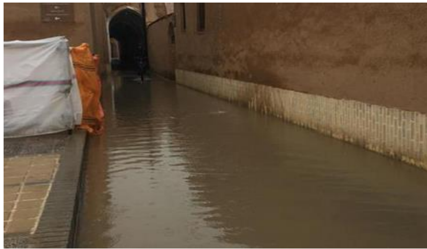
Figure.5.2. Surface Water and Poor Municipal Services (URL 27)
