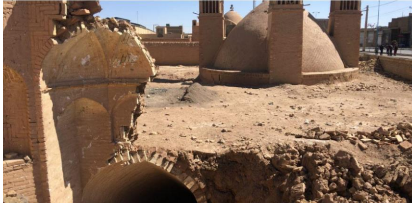
Figure.5.1. Collapsed Adobe Building, Zoroastrian Neighborhood (URL 26)
