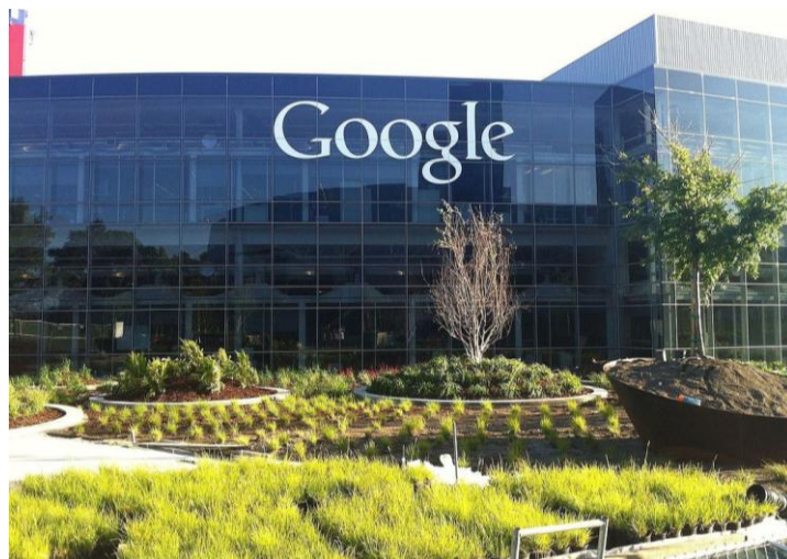
Figure 53: Outside Shot of Googleplex Company 1 (URL 48)
