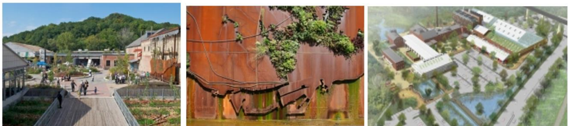
Figure 24: Evergreen Brick Works (Irvine, 2012).
