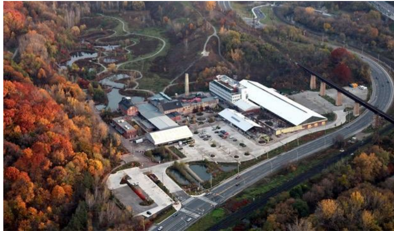
Figure 25: Evergreen Brick Works – Post-Adaptation, (Sugden, 2017)
