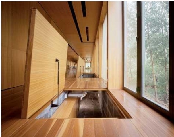
Figure 84 : Suitcase House, By Gary Chang, Hong Kong, 2001 / It Shows The Location of The Flexible of The Floor (URL:50).
