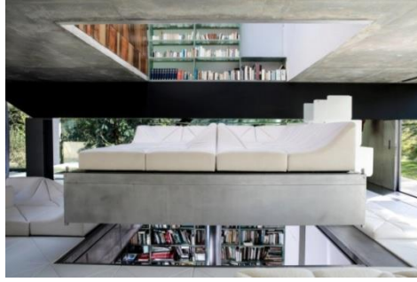
Figure 88: Villa Lemoine With Pierre Paulin’s Ensemble Dune/The Sofa is Placed on A Flexible Ceiling That Can be Moved From Top to Bottom(URL:52)
