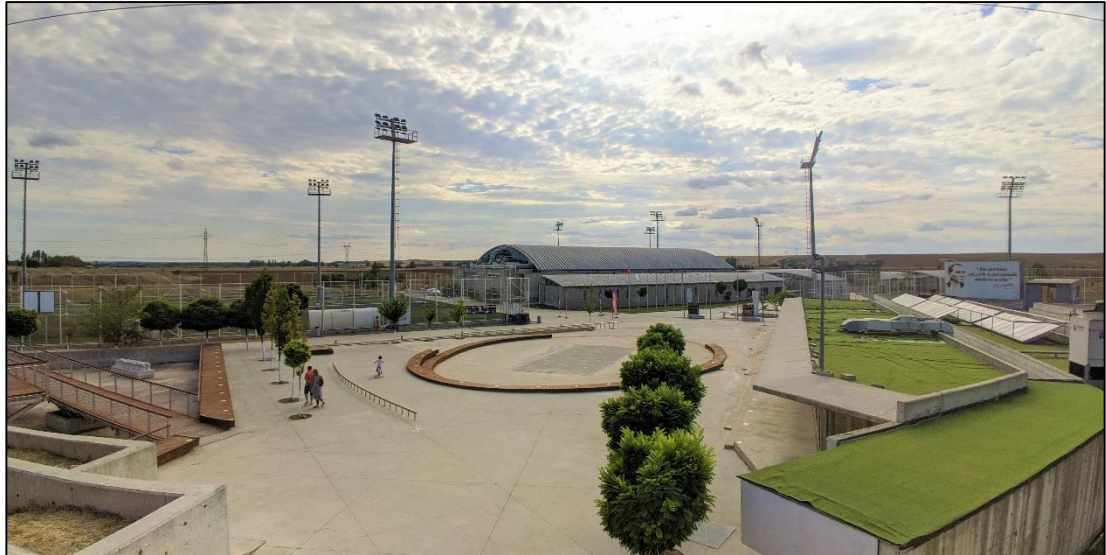
Figure 17: View from the inner courtyard of LYFA
