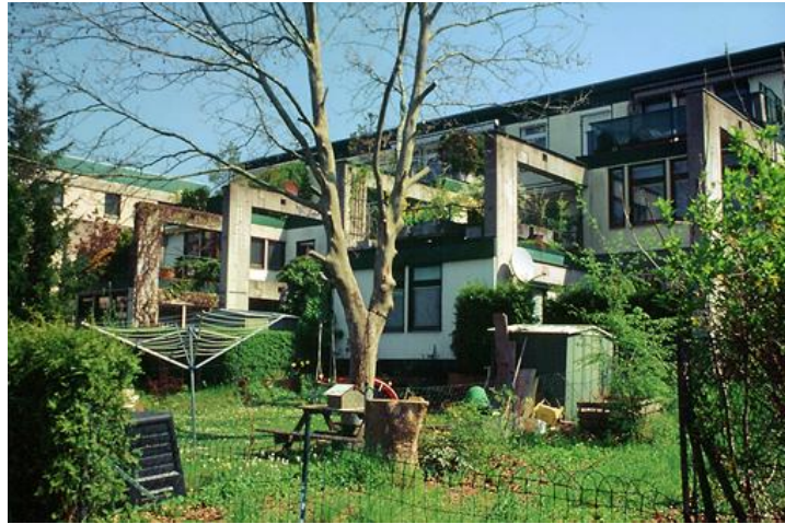
Figure 42: "Wohnen morgen" Hollabrunn, showing the relationship between structure, in April 2005 Source: (Bostenaru, 2005)
