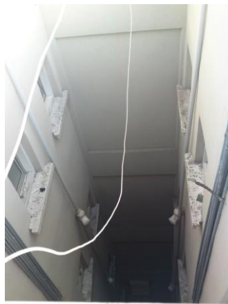
Figure 75 : top view of void between two apartments Source: (By Author, 2010)
