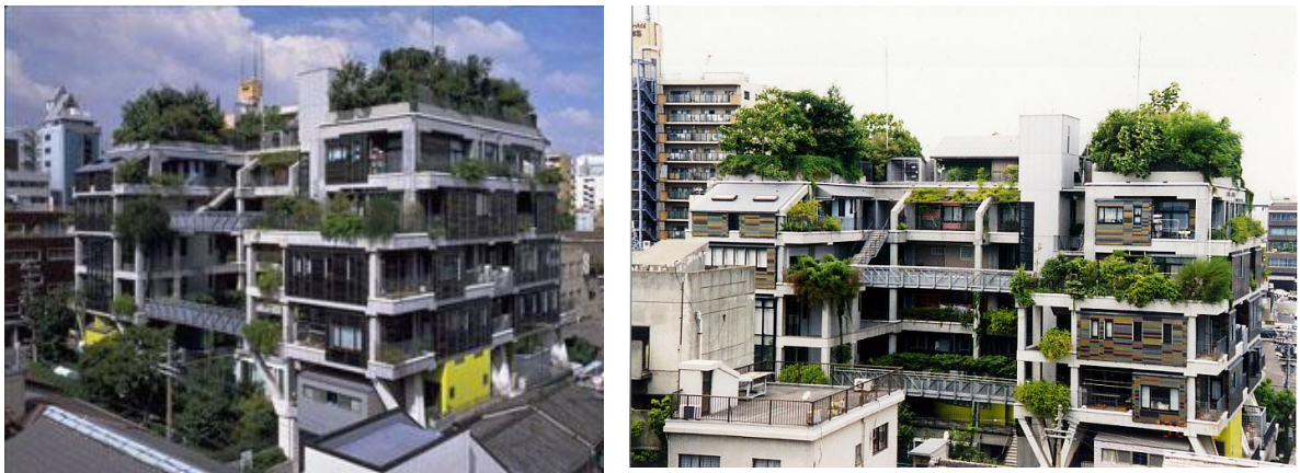
Figure 52 Image By Toyoshi Matsumoto, Osaka Gas Co. Ltd view of NEXT21 complex
