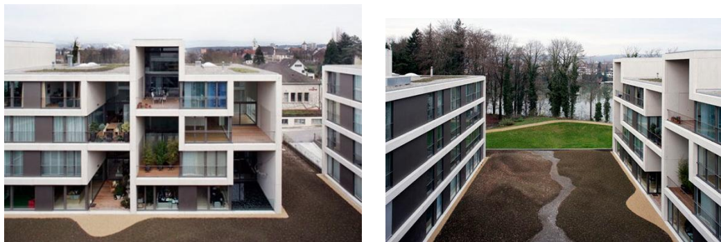
Figure 14 : Views of Tetris style housing that creates flexible living options Source: (Sejima, 2009)
