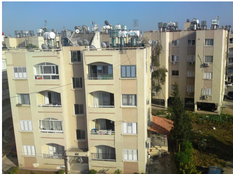
Figure 74 : View of the front facade Source: (By Author, 2010)
