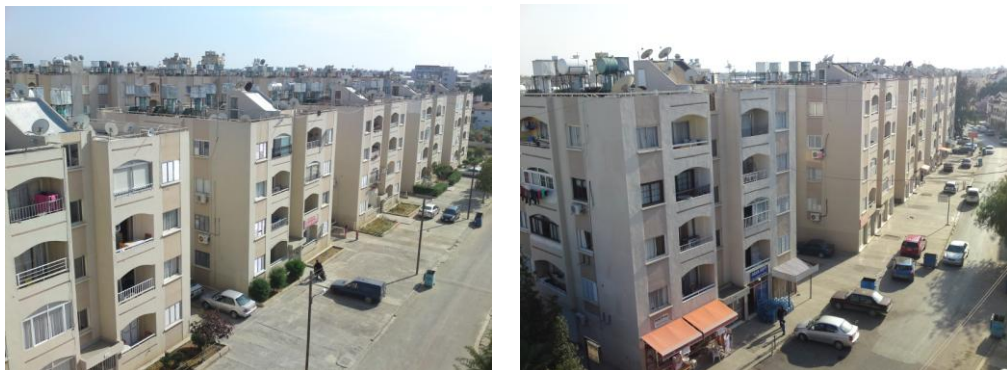
Figure 60 : Cross view of a part of a social housing area in Famagusta in 2010 Source: (By Author, 2010)
