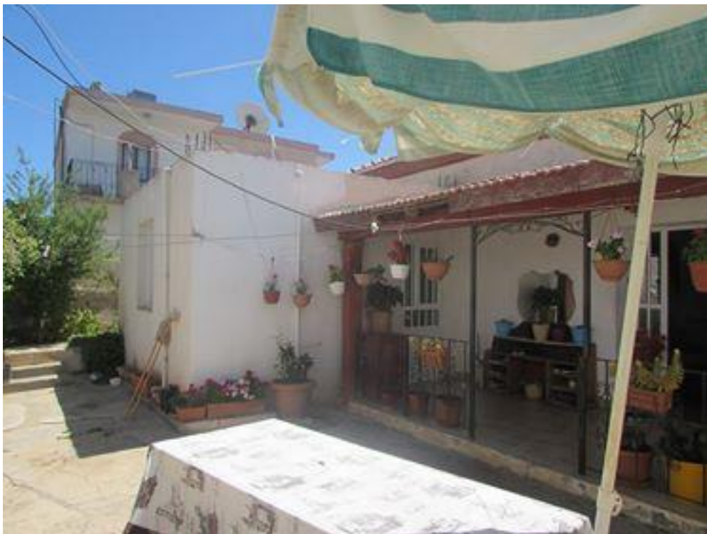
Figure 28. Showing a typical space addition of bedroom (Author,2018)
