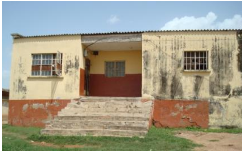
Figure 19: State Low-cost Housing typical entrance (personal archive)
