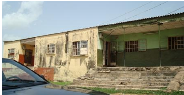
Figure 20: State Low-cost Housing entrance perspective (personal archive)
