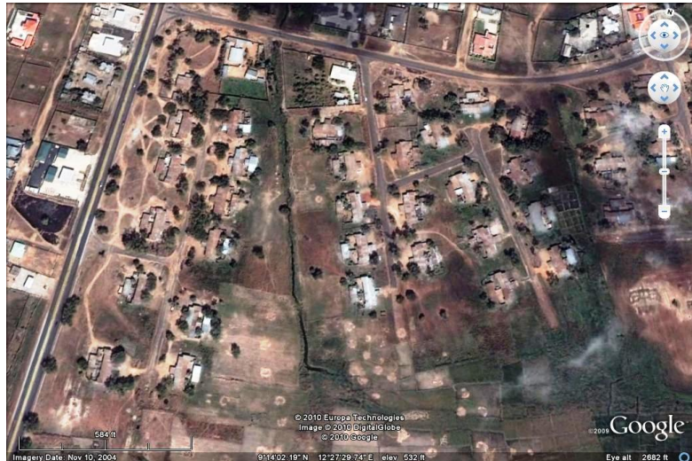
Figure 26: Aerial view showing 80 Units Housing Estate (Google earth)
