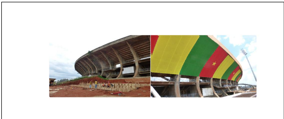
Figure 4.19: Façade made with Magic Springs Systems from PRAT SA (Roure, 2016)
