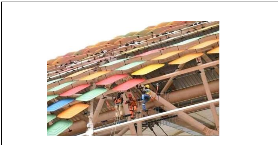
Figure 4.34: Façade Panels Installation at Olembe Stadium (Mangaleu Toukam,2023)
