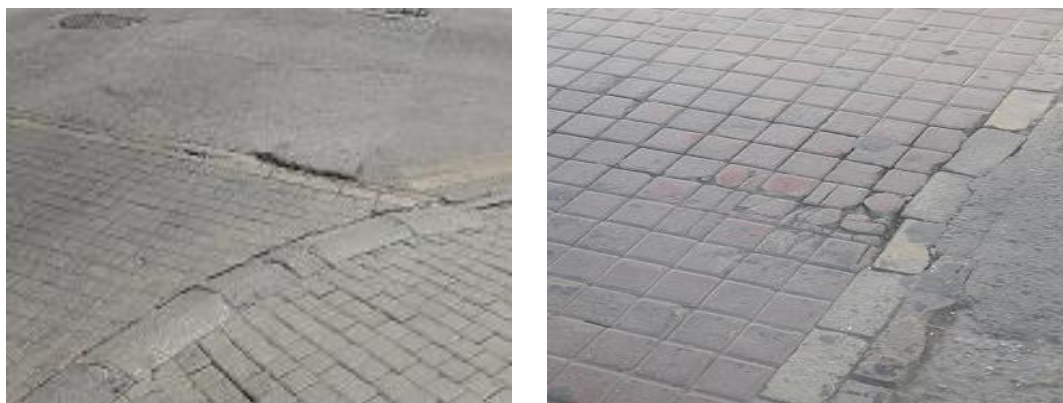
Figure 6.67: Cracked and uneven surfaces of pedestrian crossings threaten pedestrians, especially users of wheeled devices
