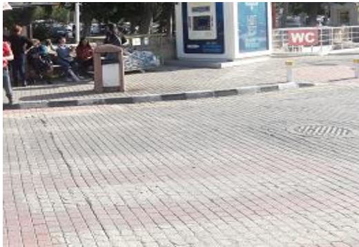
Figure 6.32: Spilled surfaces of pedestrian crossings due to traffic load and weather conditions
