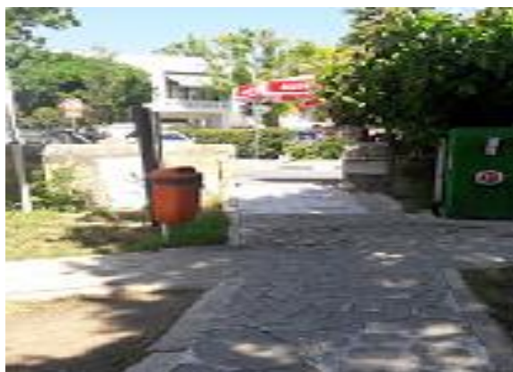
Figure 6.15: The undulated texture of pathway is troublesome for both able-bodied and disabled users
