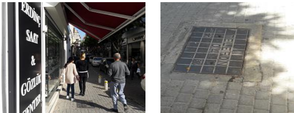
Figure 6.49: Joints between the infrastructural elements and concrete tiles are hazardous for all pedestrians, especially for those reliant on mobility aids or who experiences mobility difficulties
