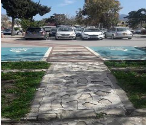
Figure 6.19: The surface texture of paving material is not suitable for all users
