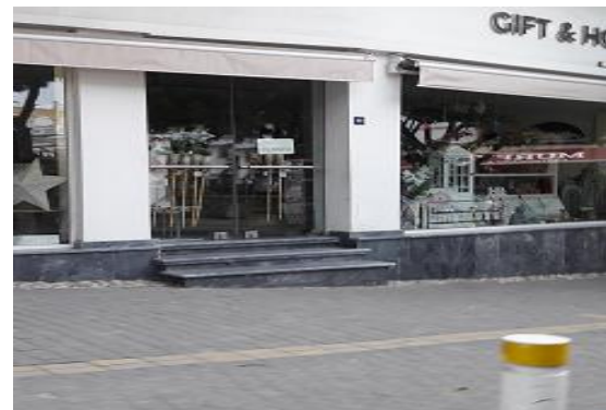
Figure 6.44: Stairs at entrance footway without any ramp design is inaccessible for wheelchair/scooter users
