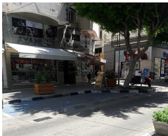
Figure 6.62: Curb-side parking facilities are not usable because of the absence of accessible curbs
