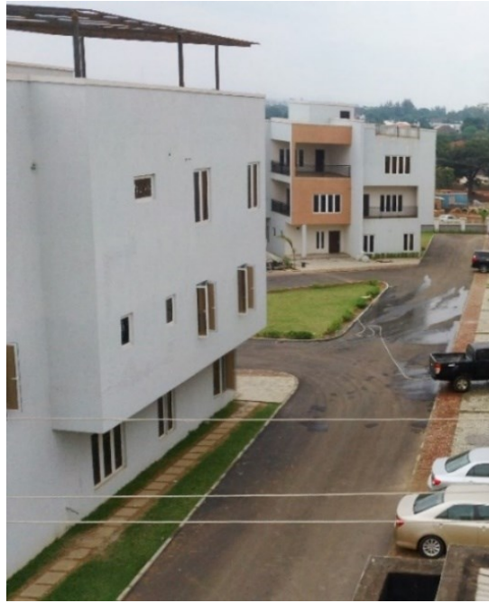
Figure 85: Narrow Windows with Poor Window to Wall Ratios in a Detached Duplex Unit in Case Study One (Ivy Homes)
