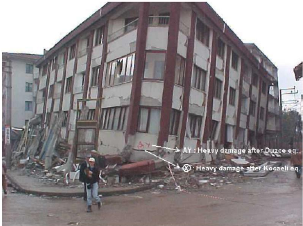
Figure 1.4: Effect of sequential earthquakes on a concrete building in Turkey (Rathje et al.2006)
