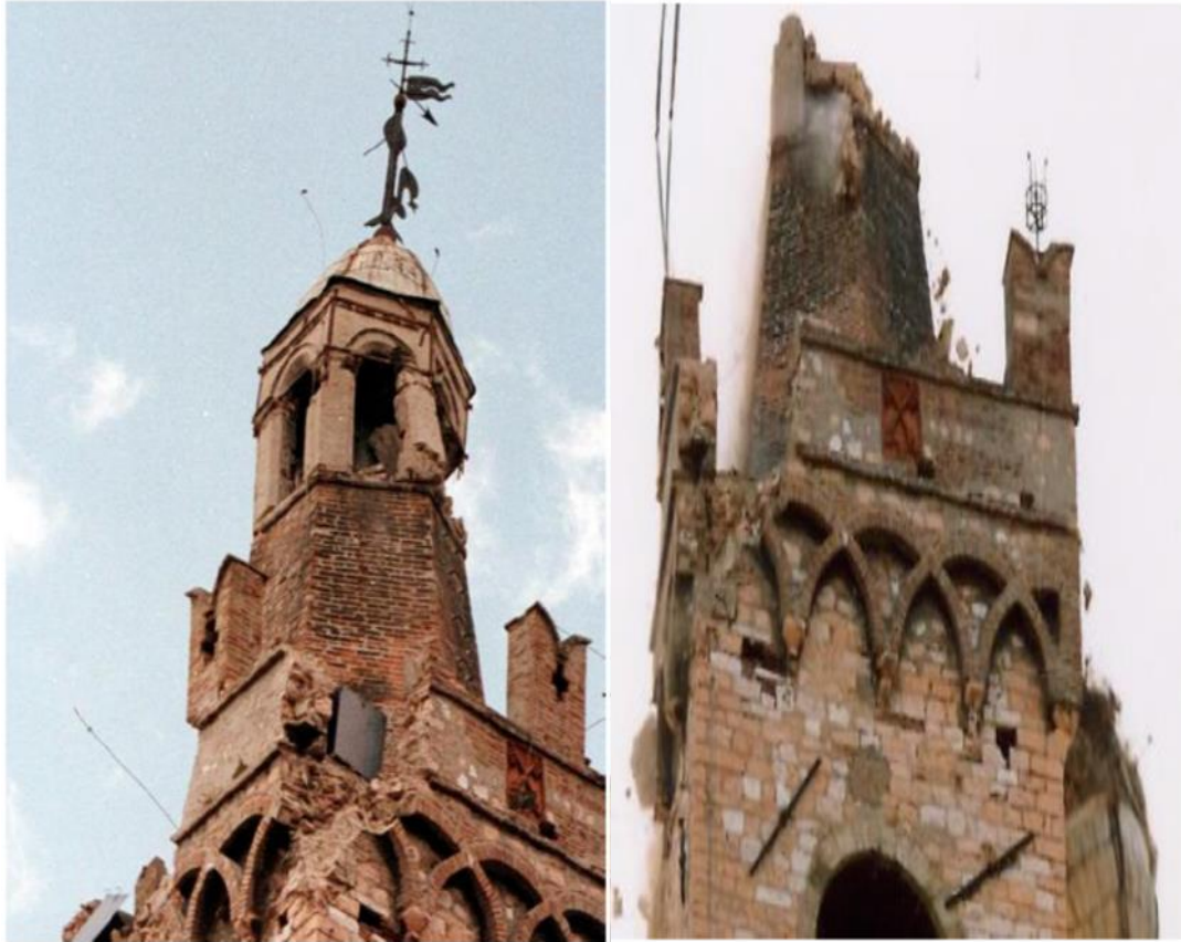
Figure 1.2: The Foligno Tower after first two sequence shock (Left). The Foligno Tower after the third sequence shock (Prete et al. 2005)
