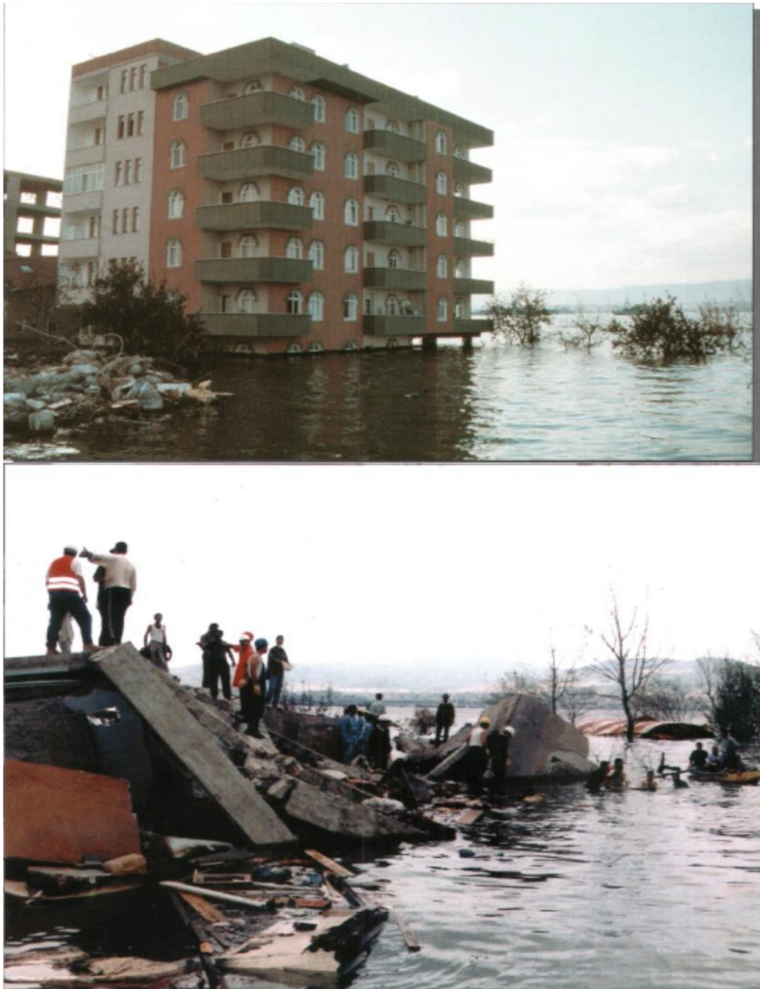
Figure 1.3: A building partially damaged from the mainshock of 1999 Kocaeli earthquake (the upper picture) and completely destroyed under the AS (the bottom picture) (photograph by Thomas L. Holzer (Gross & Phan, 2000))
