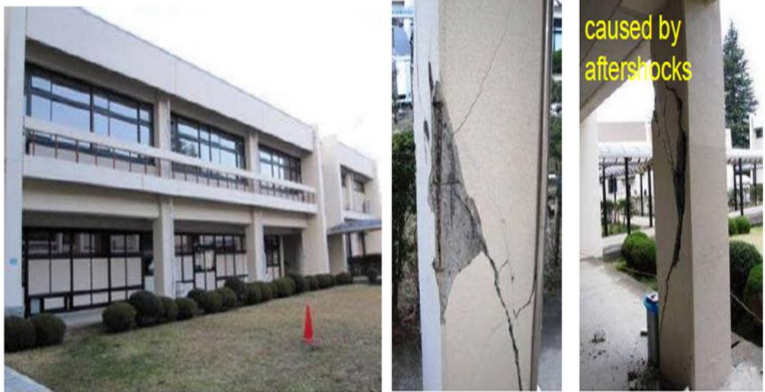
Figure 1.6: Shear cracks in a base-floor column because of ASs of the Tohoku earthquake (Nishiyama et al. 2011)
