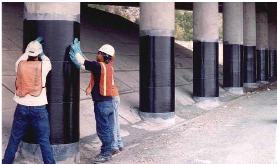
Figure 13: FRP for column [42]
