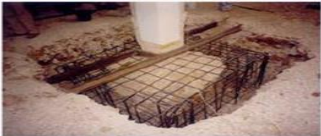
Figure 9: Jacketing of foundation [39]
