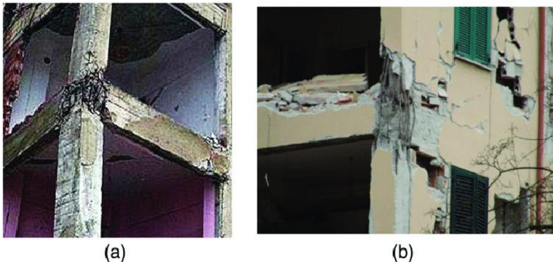
Figure 8: Failure of the corner joints of reinforced concrete structures [26]
