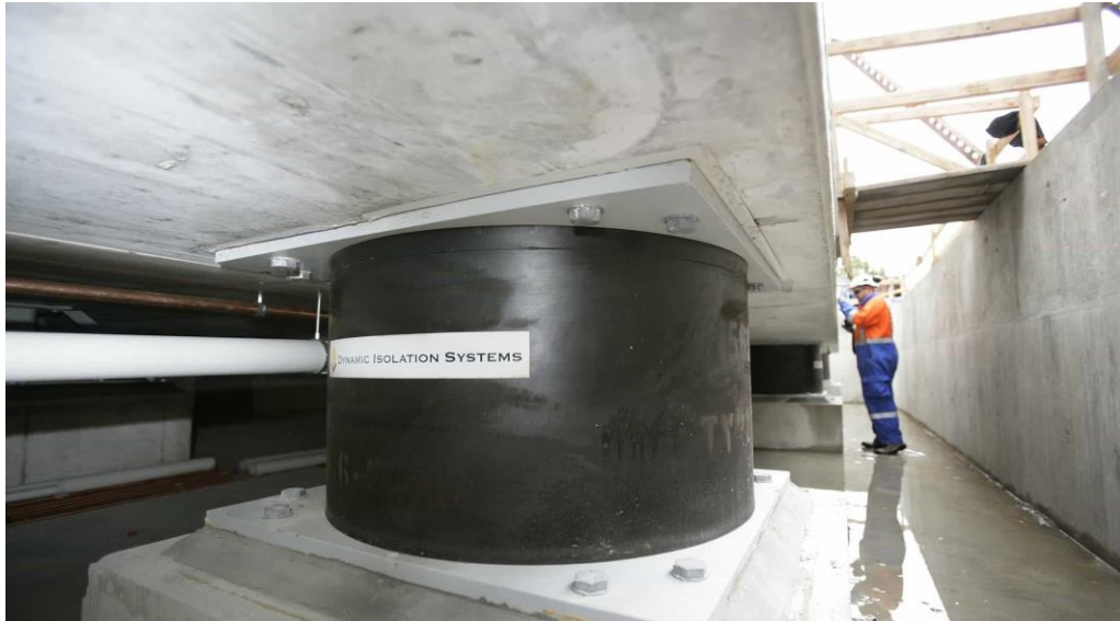
Figure 11: Base isolation for a structure from the foundation [41]
