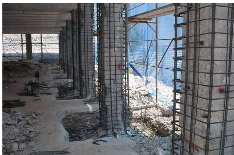
Figure 7: Column section enlargement method [28]
