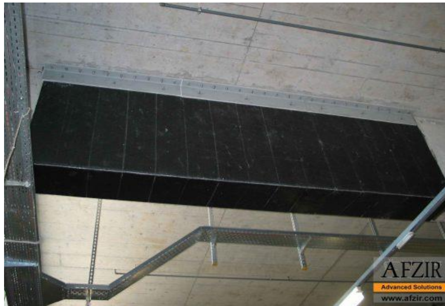
Figure 12: FRP for beam [42]
