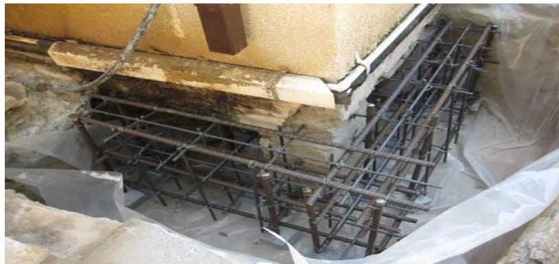
Figure 10: Underpinning of foundation if structure is not strong enough [40]
