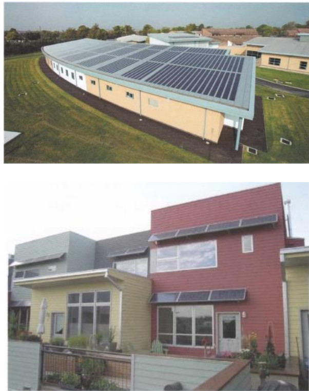
Figure 2.62: Flexible Laminates PV (Up); PV Shades (Down) (Hass, 1995)
