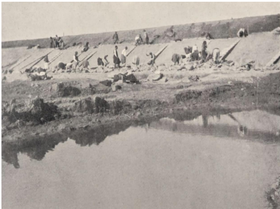
Figure 1. Construction of Kouklia Reservoir embankment (Rider, 1901).
