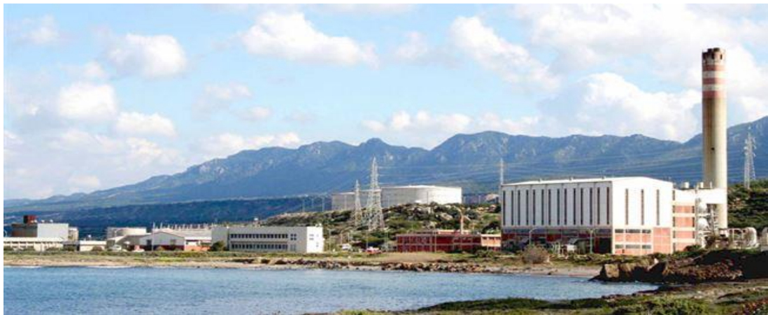
Figure 3.2: Teknecik Power Plant
