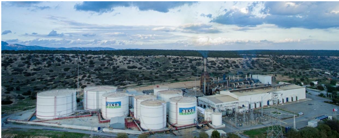
Figure 3.3: Kalecik Power Plant
