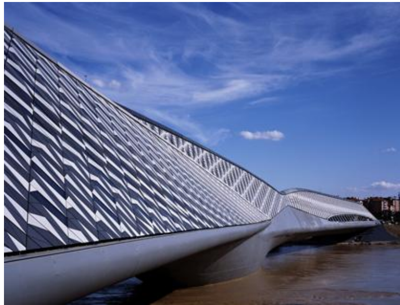
Figure 1. Zaragoza Bridge Pavilion (Rieder)
