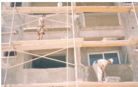
Figure 3: Unsafe scaffolding
