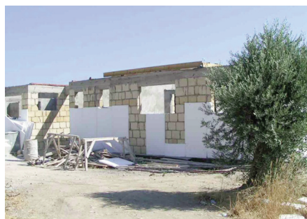
Photo 2. Detail of wall insulation. Photo taken by designer
