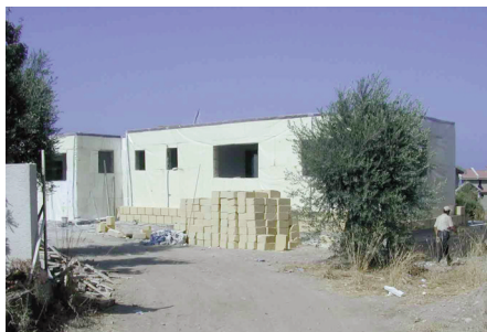
Photo 3. Detail of wall insulation. Photo taken by designer.
