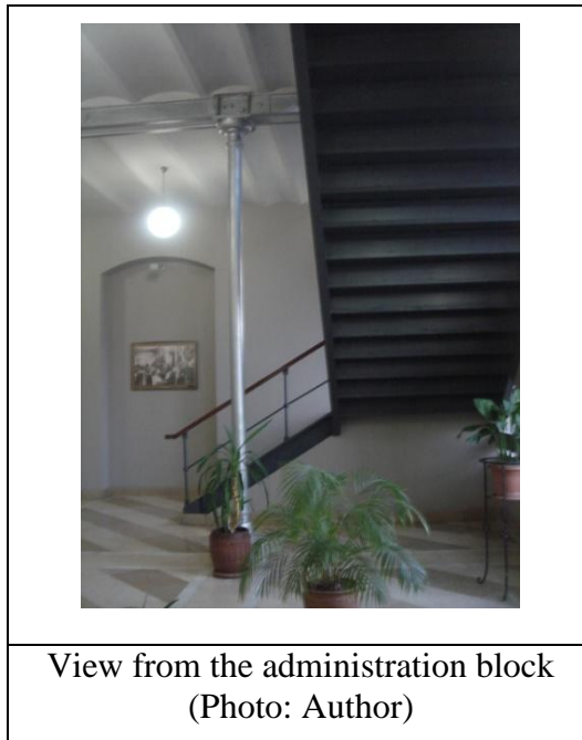
Figure 72. Additional floors supported with steel columns
