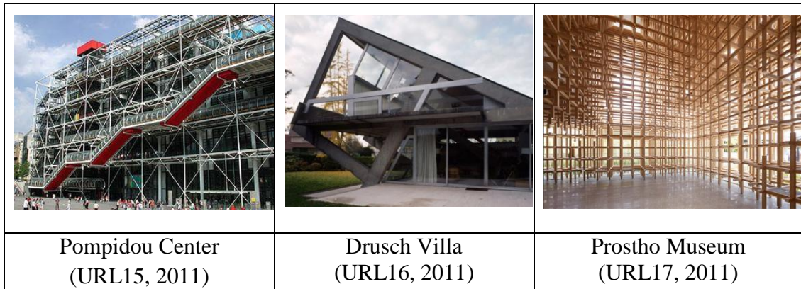
Figure 34. Example of steel, reinforced concrete and timber frame respectively
