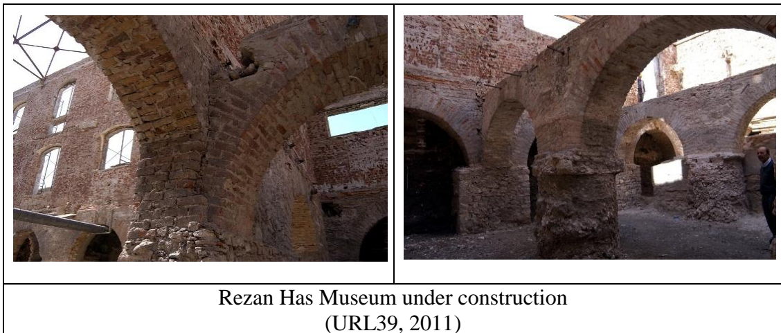
Figure 73. Construction process of the museum block
