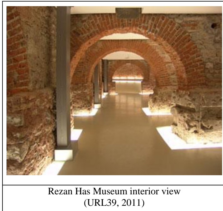
Figure 74. Steel columns are placed in the museum
