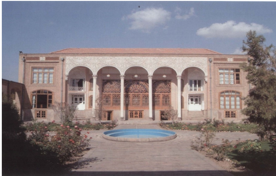
Figure 51: One of the vernacular buildings (Behnam House) in Tabriz which has central courtyard, but no summer living quarter (Kleiss.W, 1995)
