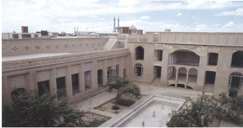
Figure 38: Northern and western side of the courtyard of Sigari's (University, 2005)
