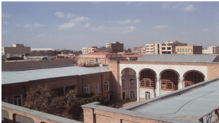
Figure 53: One of the vernacular buildings (Gadaki House) in Tabriz which has central courtyard, but no summer living quarter (Kleiss.W, 1995)
