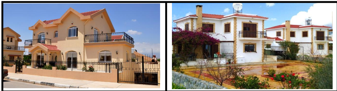
Fig 4.8. No strategies or elements were used in windows or terraces for providing shadow during summer. The terraces and balconies are open to sky
