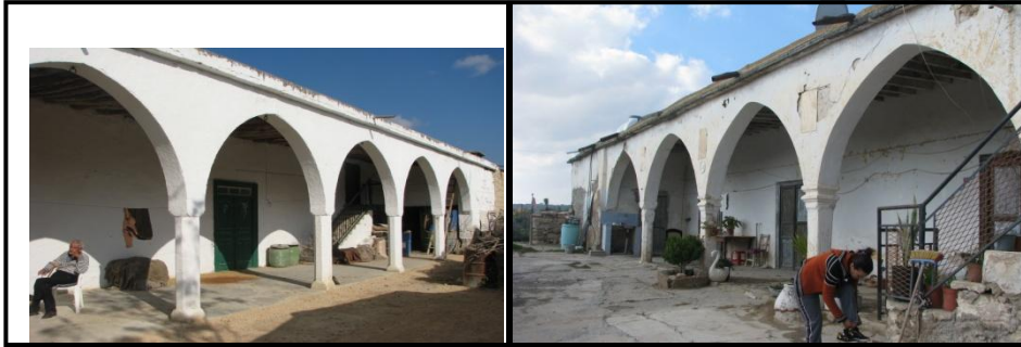
Fig 3.10.rural houses with outer hall ( Author, 2011)
