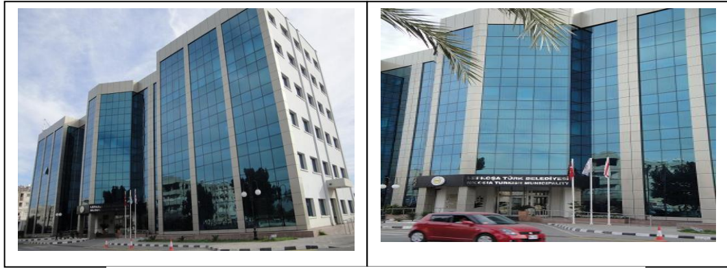
Figure 4-15: View of Lefkoşa Türk Belediyesi Building
