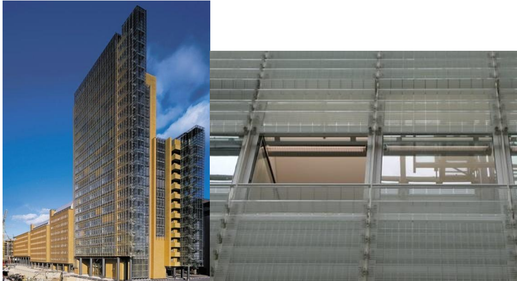
Figure 2-36: Debis-Building; Located in Berlin, Germany; in 1998; Architect Renzo Piano. a) View of the facade (URL 48); b) detail of the DSGF system (URL 49); the Window system is used with timber made louver blinds in the void between interior facade and exterior skin. The facade is composed of prefabricated terra-cotta elements and glass. The second skin of the facade reduces ND, even when designed for maximum transparency. The interior spaces are equipped with openable windows, but a mechanical system controls the ventilation as well (IBUS, n.d).
