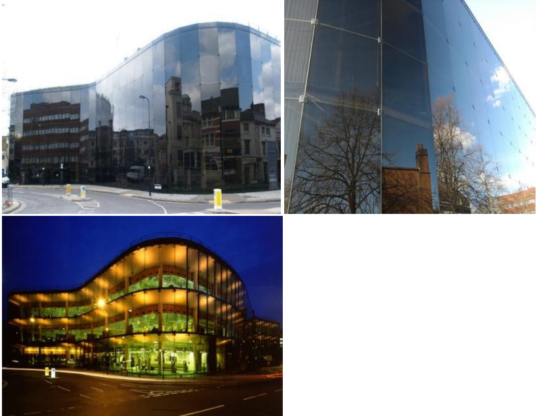
Figure 2-8: Willis Faber & Dumas Building; in Ipswich, by Foster and Associates, 1972 (URL 15; URL 16; and URL 17).
