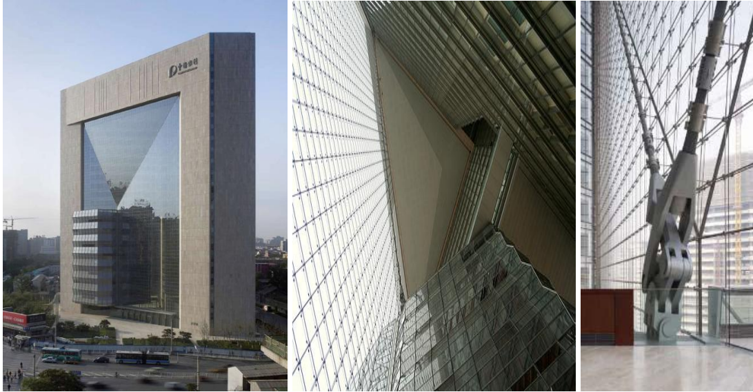
Figure 2-9: New Beijing Poly Plaza; by SOM architect, 2007, China. Cable net support system with rocker arm detail (right) (URL 18; URL 19; and Patterson, 2008: 241).
