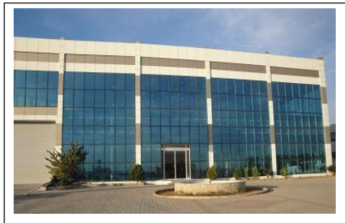
Figure 4-25: View of Saray Aliminyum LTD Building
