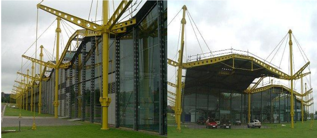
Figure 2-20: View of Renault Center; by Foster and Partners in Swindon, England, built in 1982 (URL 31, and URL 32).
