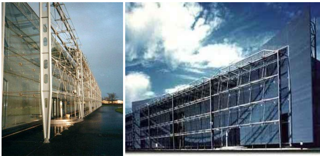
Figure 2-23: Suspended GF of Banque Populaire de l'ouest et de l'Armorique; located in Rennes, France, built in 1989 by architects Odile Decq and Benoit Cornette, with RFR, and Peter Rice. In the suspended GF the upper row of glass panes is attached to the roof edge via spring assemblies at the center. The next rows are suspended below them via cross-shaped bolted fixing. The types of glass used are toughened single panes and insulating glass panes. The facade provides ND, maximum transparency with less visual barriers (Compagno, 1999: 99), (URL 35; URL 36).
