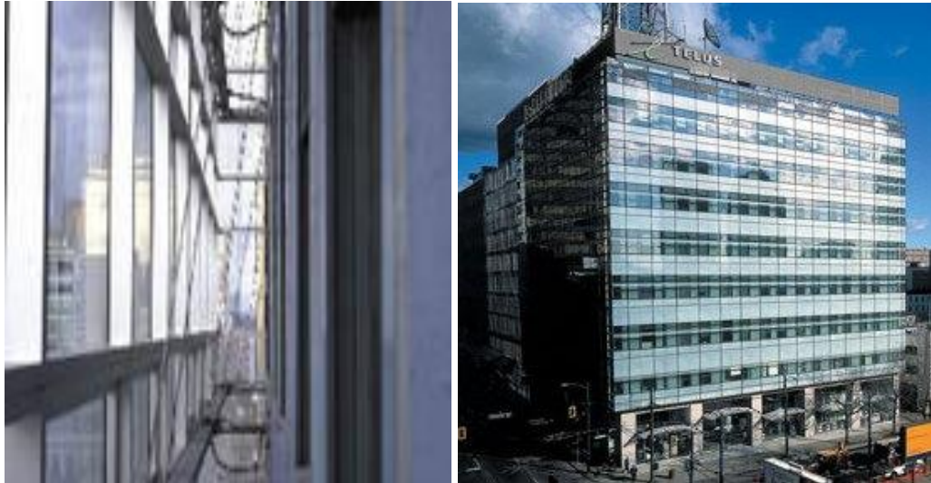
Figure 2-34: Telus-William Farrell Building; in 2000, located in Vancouver, British Columbia; Busby and Associates Architects. a) View of the facade (URL 46); b) View of the cavity; (URL 47). The facade is the first triple-skinned system in Canada. Suspended from the existing building face approximately 90cm, a new double glazed fritted glazing system, including openable windows, was hung. The air space acts as the main mechanism to help regulate the building's internal temperature, contributing in both cold and warm weather. The cavity is both naturally and mechanically ventilated in which in winter it is closed from top and bottom and it insulates the building. In summer the cavity is open and in order to increase the air movement in the cavity, mechanical fan might be used (Gilson, n.d).
