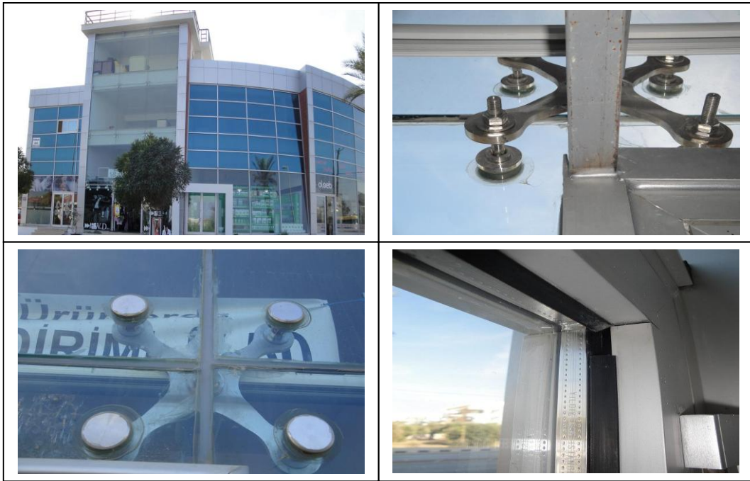
Figure 4-29: View of Ofton Building
