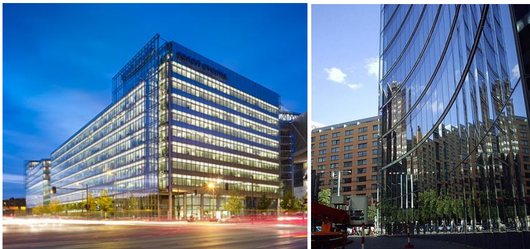
Figure 2-22: GF of Sony Center in Berlin; Murphy/Jahn Architects; 1992-1999. Facade is supported by glass fins, also for wind bracing (URL 34; URL 35; and Compagno, 1999: 22).
