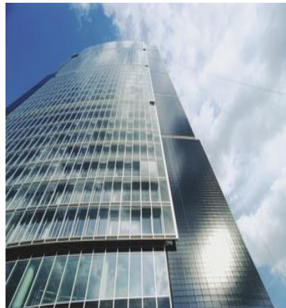
Figure 2-31: Example of Shaft-Box DSGF; ARGA Insurance, Dusseldorf; Architects: Rhode Kellermann Wawrosky and Partners (RKW) in cooperation with Foster and Partners (URL 45).
