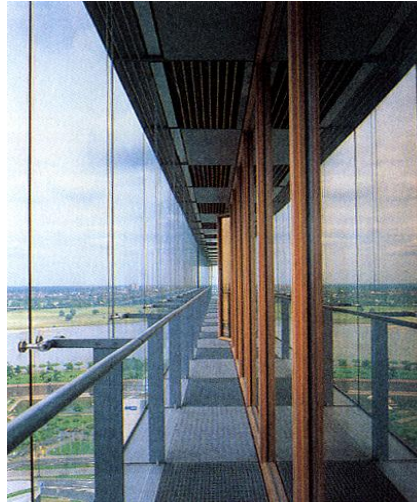
Figure 2-30: Example of Corridor DSGF; Dusseldorfer Stadttor Building, Dusseldorf, Germany; Architects: Petzinka Pink and Partners (URL 44).
