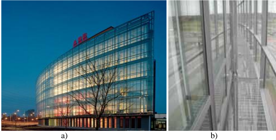
Figure 2-12: DSGF of ABB Business Center; in Sweden, by Architect: BSK after ideas from Archus-Arosia, in 2002: a) View of ABB (URL 23); b) View of the cavity (Poirazis, 2004: 134).
