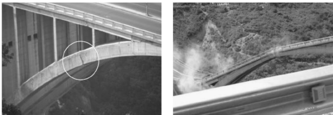
Figure 2.6: Collapse of Viaduct 1 concrete arch bridge [13] Left: east arch rupture (January 5, 2006); Right: Bridge collapse (March 19, 2006)
