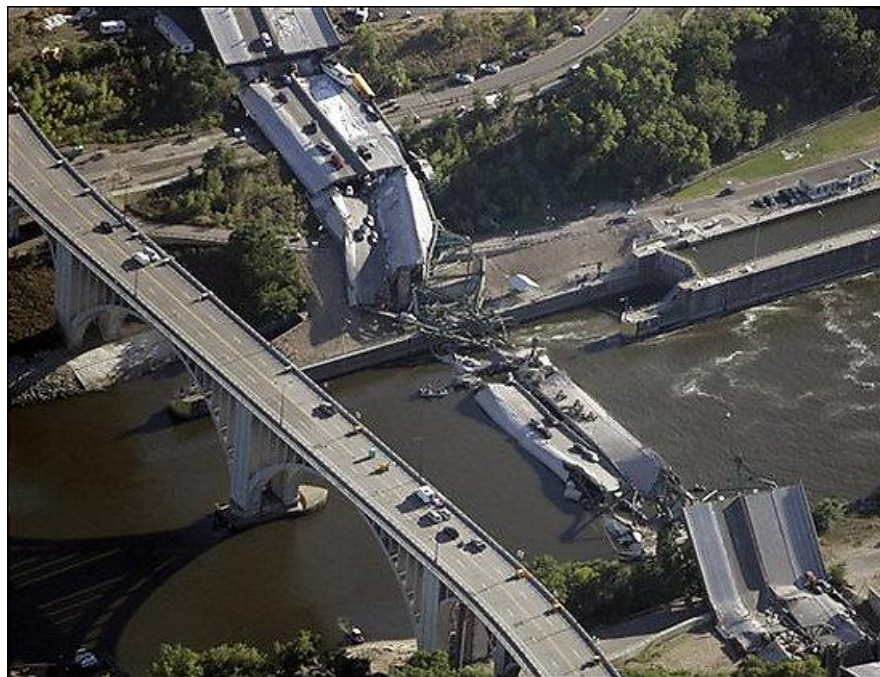
Figure 2.10: View of the collapsed I-35W bridge [3]
