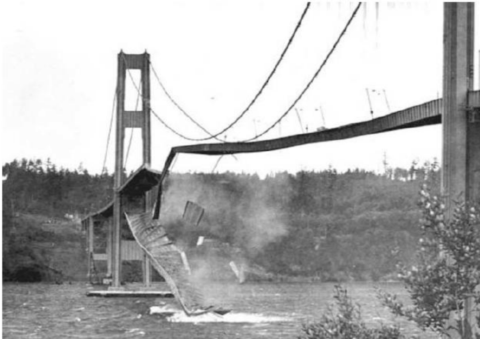
Figure 2.5: Tacoma Narrows Bridge collapse [15]
