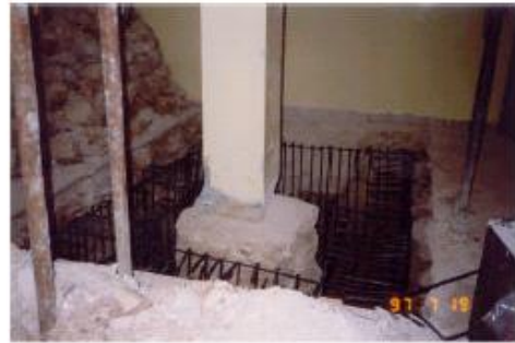
Step#2 hardening the surface and installing the dowels.
