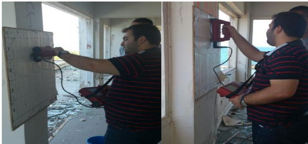
Figure 62. Reinforcement details scanning by Ferroskan.
