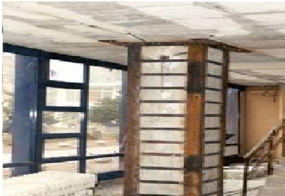
Figure 32. Increase strengthening by Steel angles.
