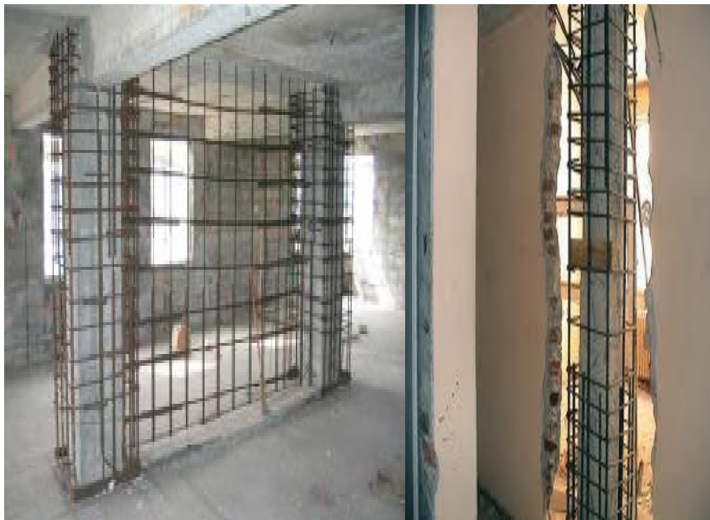
Figure 41. Adding Shear walls and Columns.
