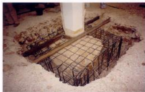
Step#4 Completing the jacket.
