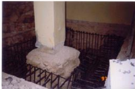
Step#3 Installing the main steel.
