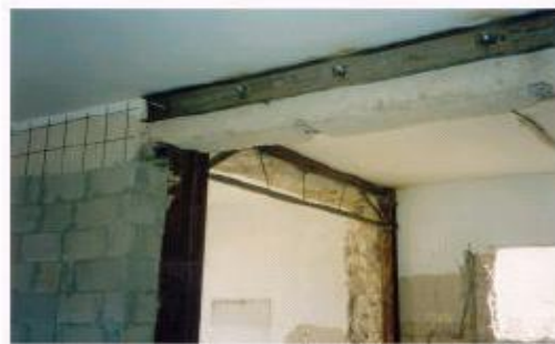
Strengthening by steel plates.
