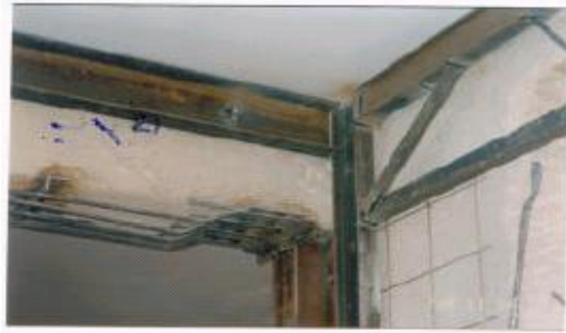
Strengthening a beam and Slab.
