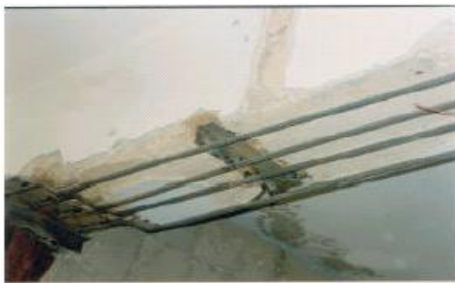
Jacketing a beam by increasing bars and cross section.
