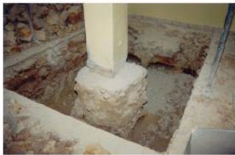
Step#1 Excavating around the footing.
