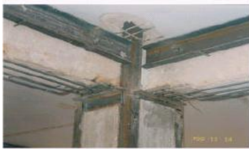
Strengthening a beam , slab and column.
