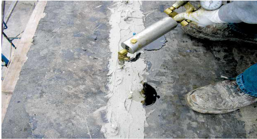
Figure 22. Crack repairing used Epoxy grout [27].
