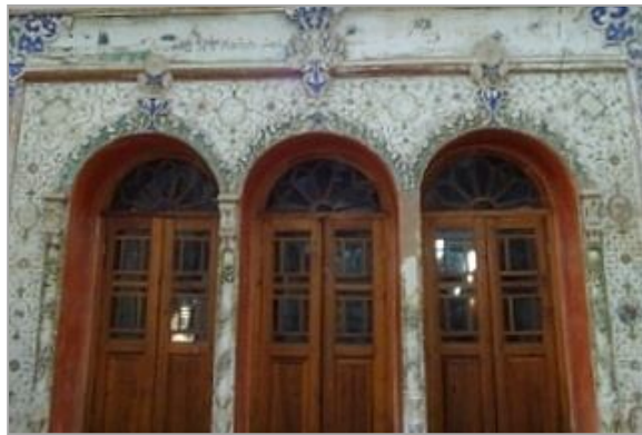
Figure 39: Se Dari (three door room) of an Iranian traditional house in Kashan, Iran.
