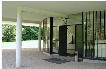
Figure 12: Pilotis (supporting columns) (Corbusier, 2001).
