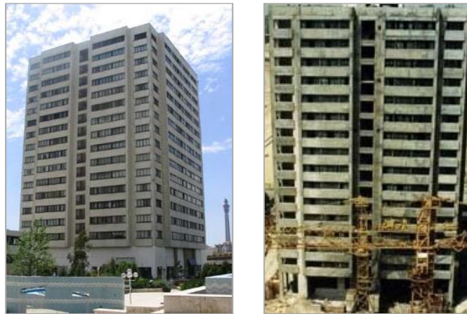
Figure 58: Usage of industrialized method, prefabricated elements in construction, In second period (1941- 1979) (Vanak park Co., 1978).
