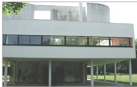
Figure 8: Applying white color and emphasis of horizontal line in façade of one modern building (Corbusier, 2001).
