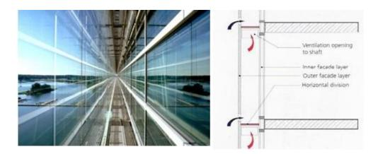
Figure 4: Shaft Box Window (Schulze, Eicker, 2013)
