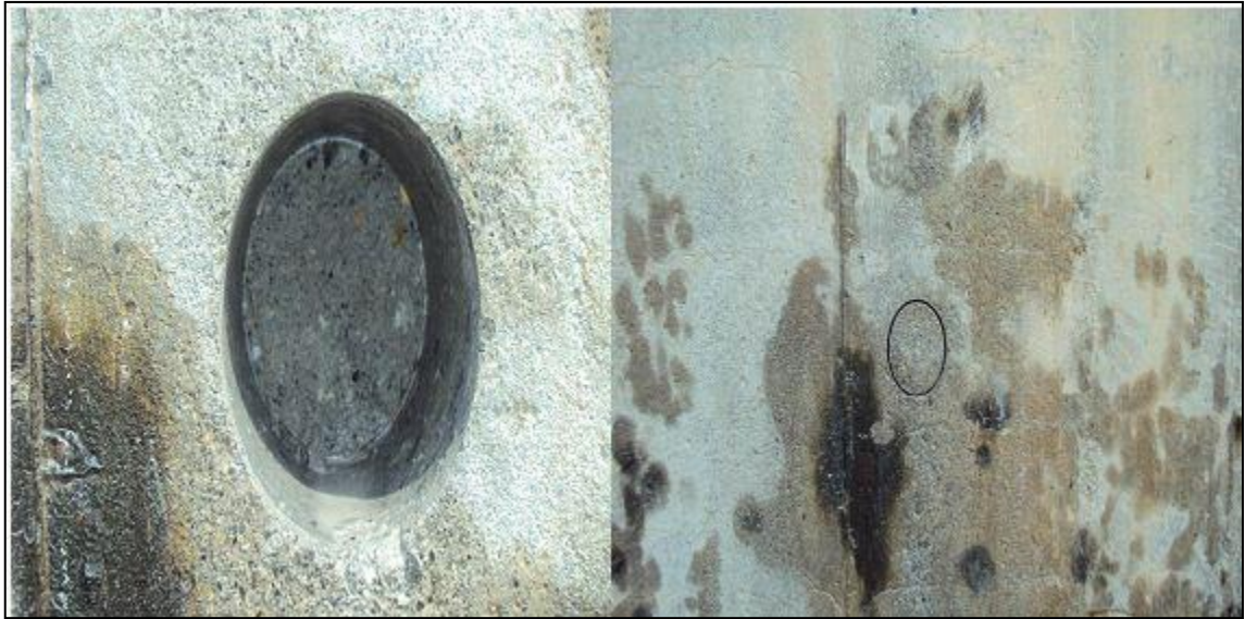
Figure 5.3: Sample Core Drilled
