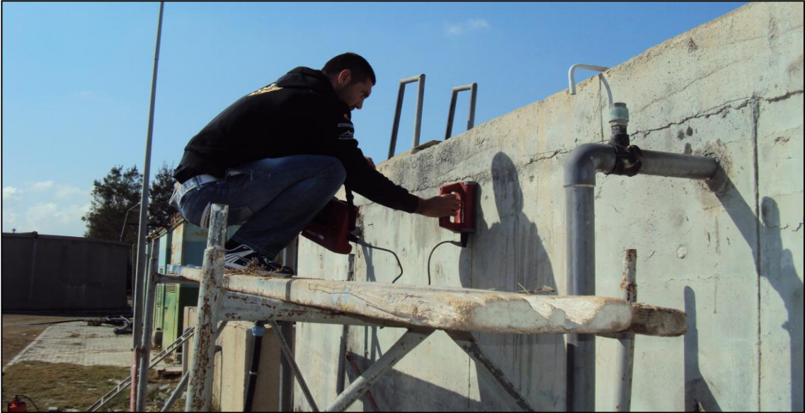
Figure 5.1: Determination of Core Sample Location
