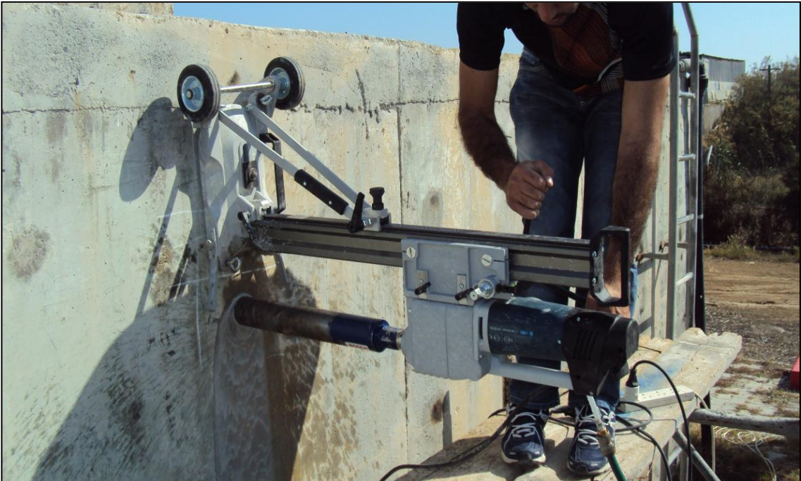
Figure 5.2: Sampling Core Operation
