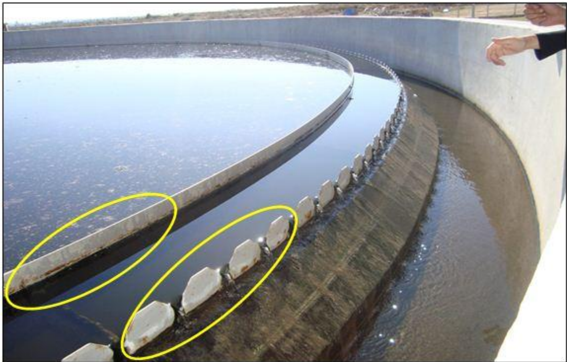
Figure 4.2: Rust Layer on the Secondary Tank
