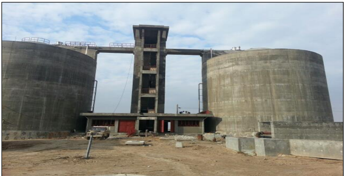
Figure 3.4: Digester Tank in Baquba-Iraq WWTP
