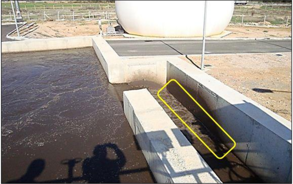
Figure 4.4: The Effect of Microorganism on Concrete Surface in Main Lagoon
