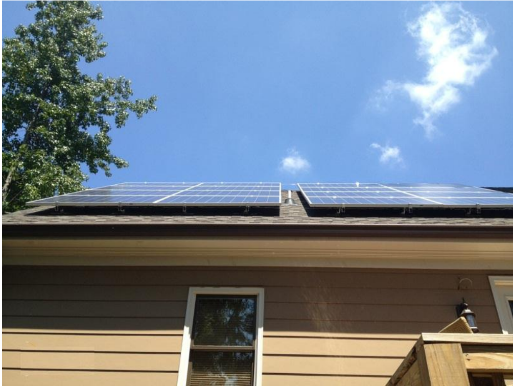
Figure 18: Residential PV Panels Install in San Giovanni In fiore, Italy.
