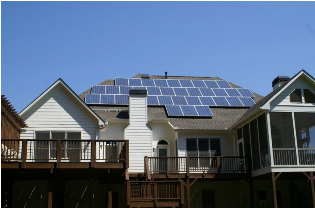
Figure 19: Residential PV Panels Install in San Giovanni In fiore, Italy.
