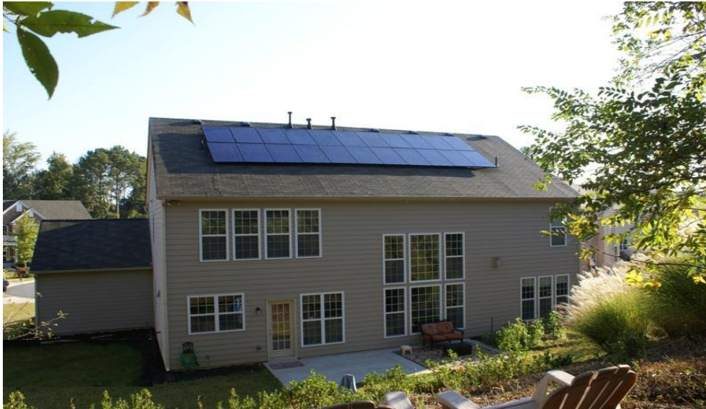
Figure 14: Residential PV Panels Install in San Giovanni In fiore, Italy.
