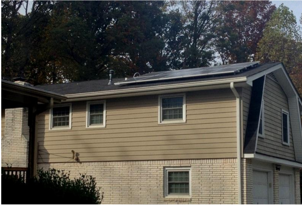
Figure 16: Residential PV Panels Install in San Giovanni In fiore, Italy.
