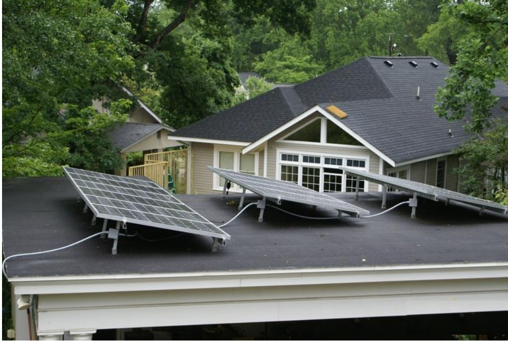
Figure 20: Residential PV Panels Install in San Giovanni In fiore, Italy.
