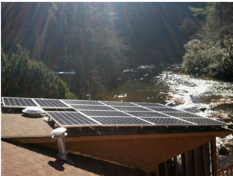
Figure 23: Residential PV Panels Install in San Giovanni In fiore, Italy.
