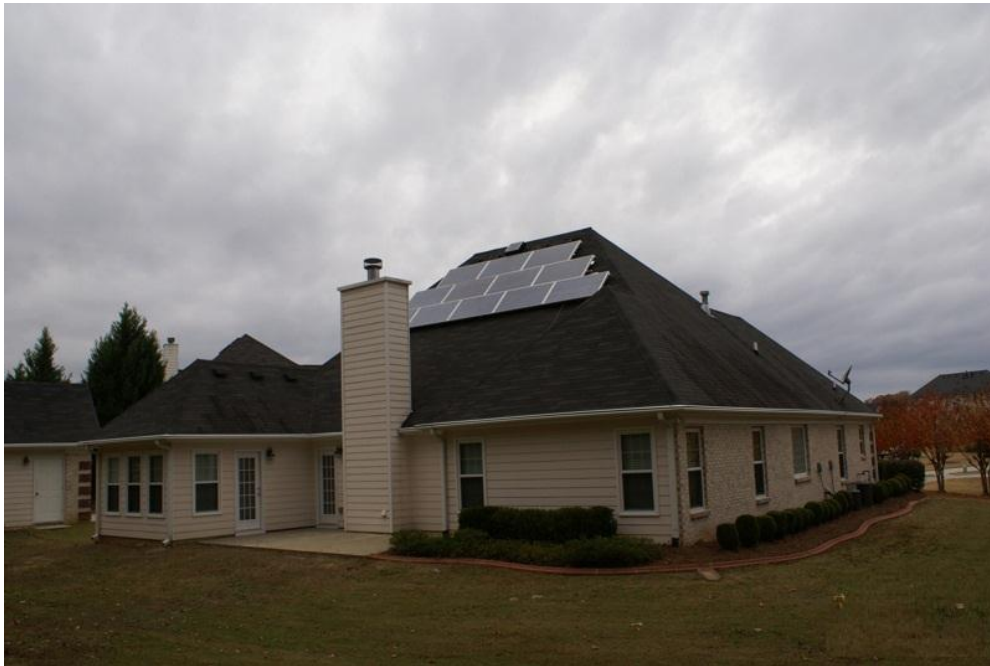
Figure 22: Residential PV Panels Install in San Giovanni In fiore, Italy.
