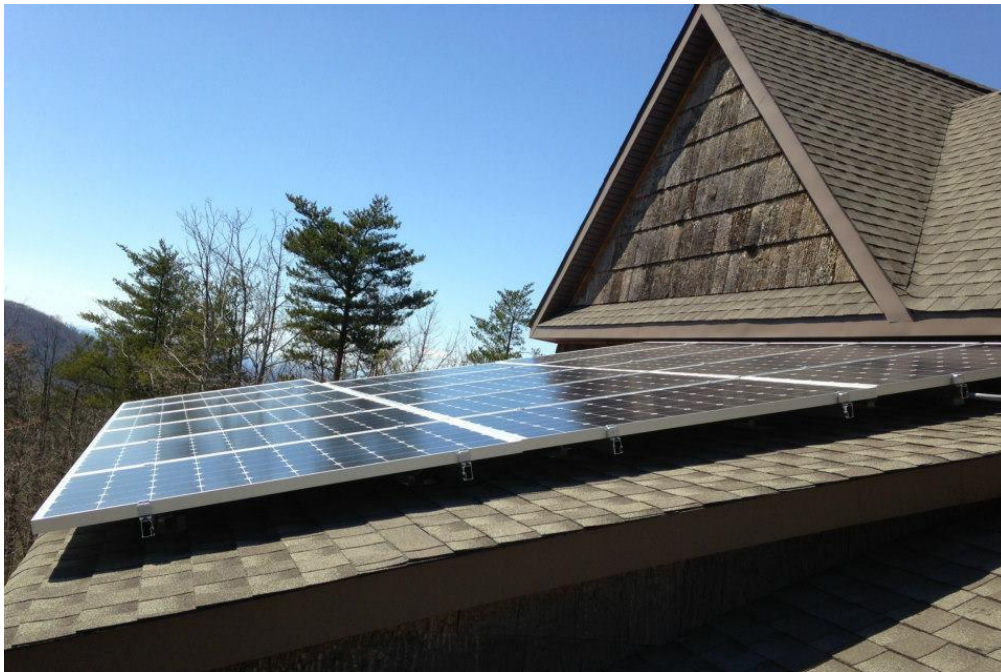
Figure 17: Residential PV Panels Install in San Giovanni In fiore, Italy.
