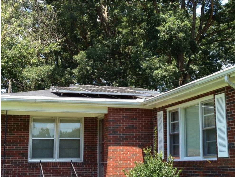
Figure 24: Residential PV Panels Install in San Giovanni In fiore, Italy.
