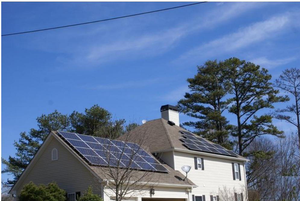
Figure 21: Residential PV Panels Install in San Giovanni In fiore, Italy.
