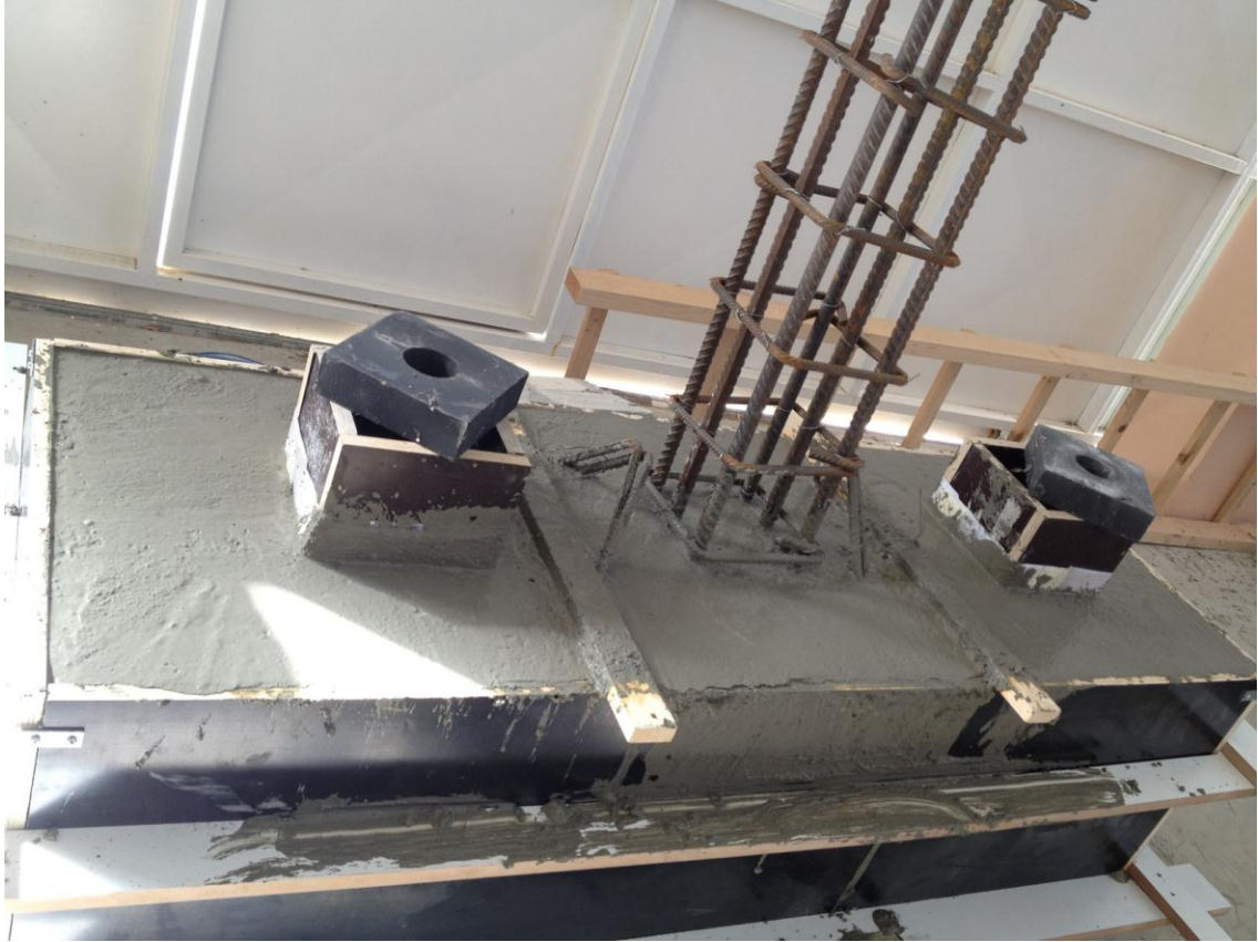
Figure 3-24: Finished footing surface
