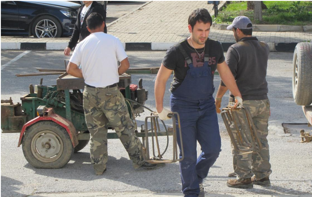
Figure 3-7: Bending the stirrups
