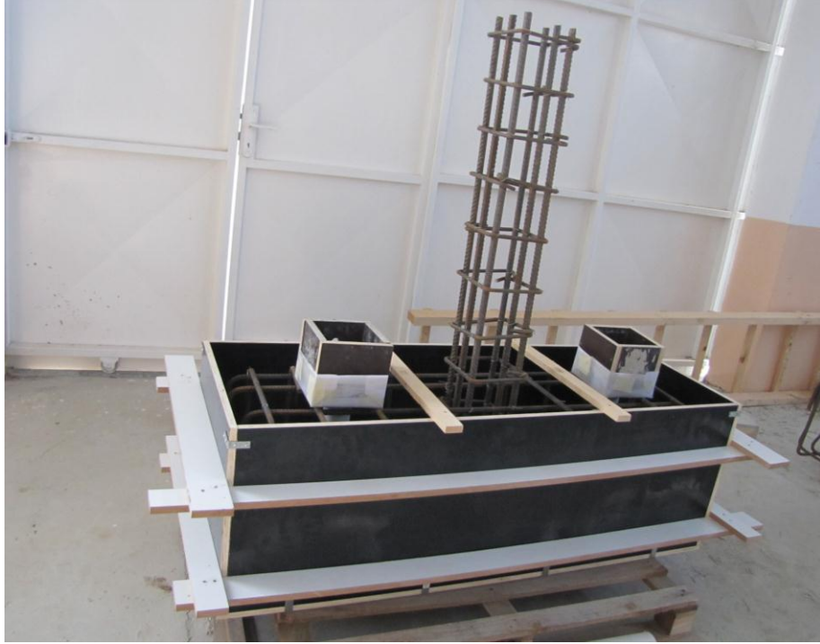
Figure 3-14: Timber supports around the main formwork
