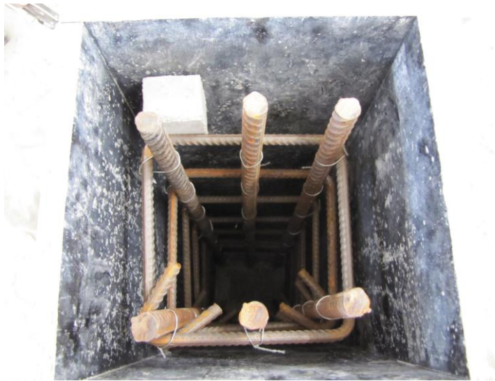
Figure 3-17: Adjusting the concrete cover for column
