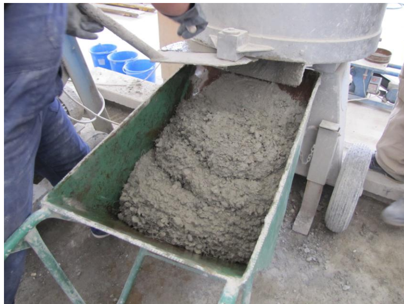
Figure 3-21: Using wheelbarrow to transfer the concrete
