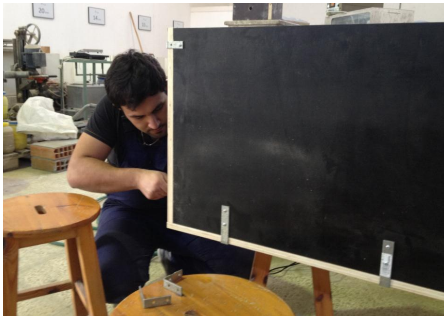
Figure 3-12: Using corner staples to fix the formworks part
