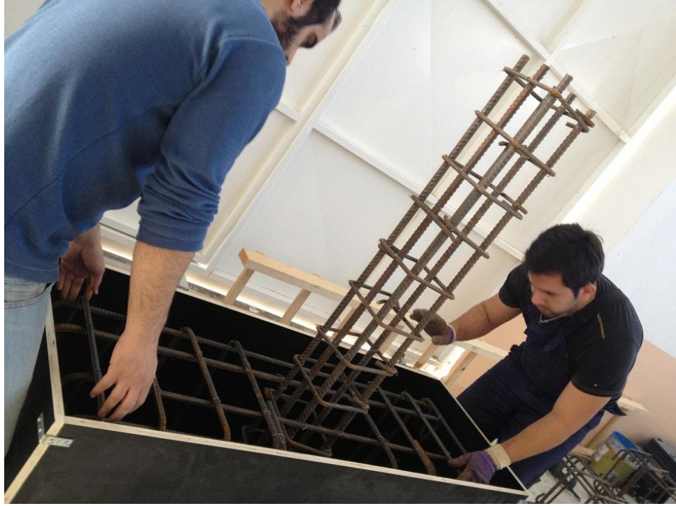
Figure 3-13: Placing the steel bars in the formwork
