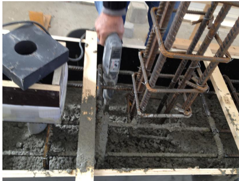
Figure 3-23: Vibrating the concrete with poker vibrator
