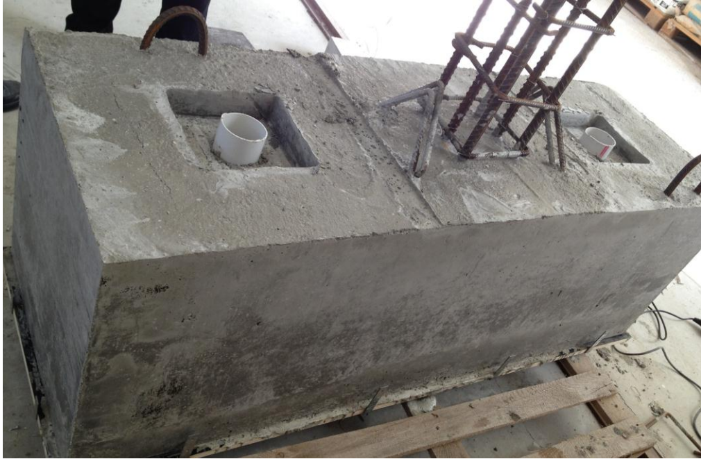
Figure 3-27: After removal of the formworks
