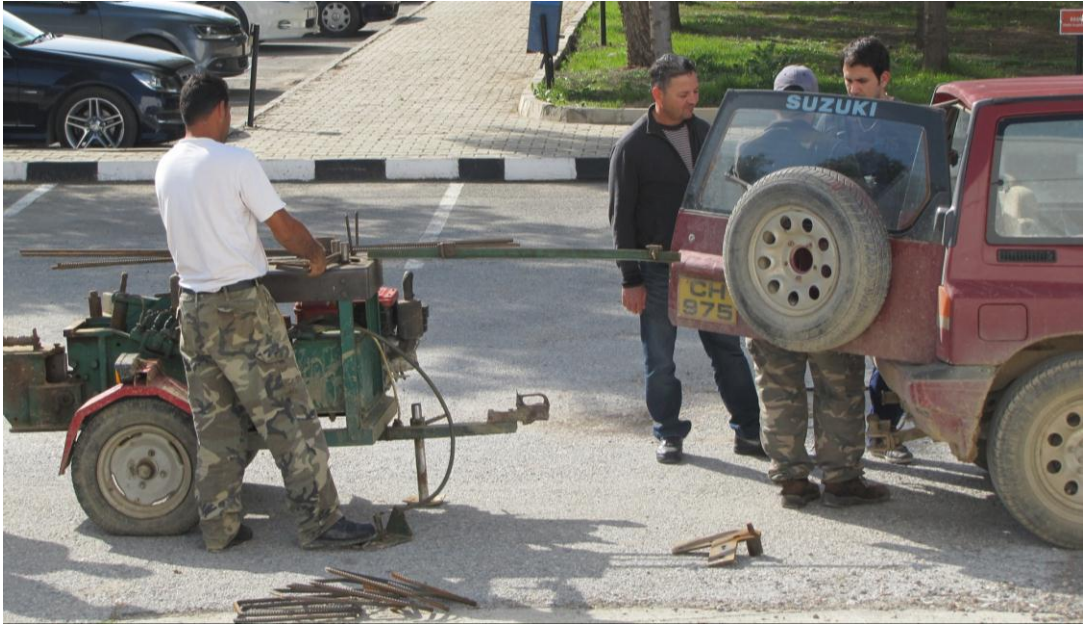
Figure 3-6: Cutting the steel bars
