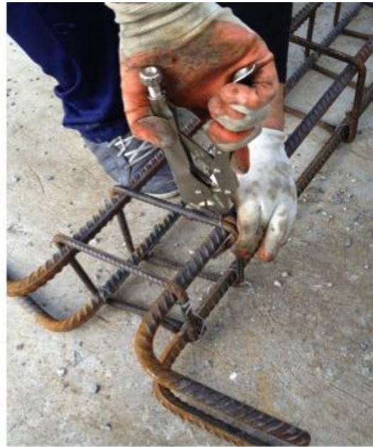
Figure 3-8: Bent bars and stirrups
