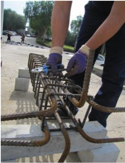
Figure 3-9: a) Fixing the main bars. b) Fixing the stirrups
