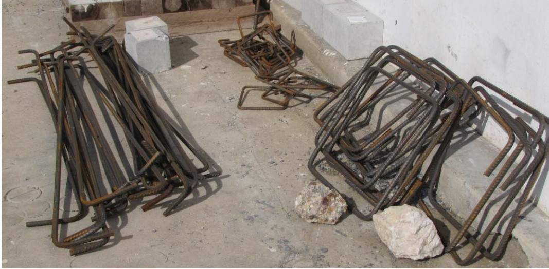
Figure 3-8: Bent bars and stirrups
