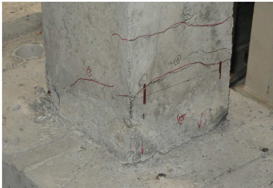
Figure 4-8: Ultimate cracks in tension side of second column (1.5% fiber)
