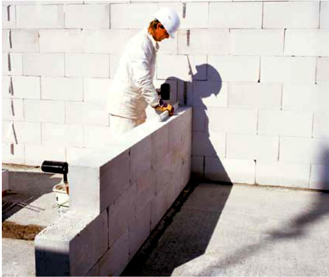
Figure 2.9: Construction of masonry wall with AAC blocks [11]
