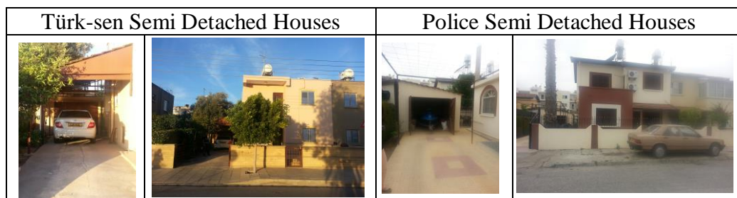
Figure 136. Addition of Garage in Police and Türk Sen Semi Detached Houses
