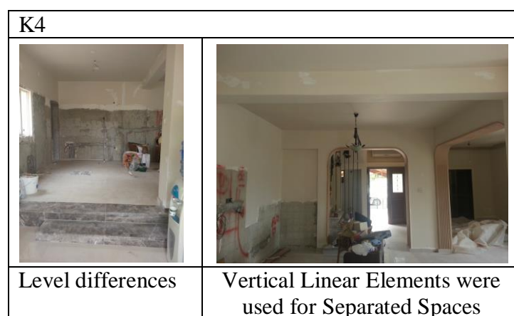
Figure 117. Level Differences and Vertical Linear Elements in Government Social Houses in Göçmenköy
