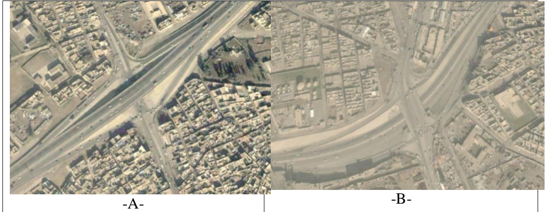
Figure 2-5: Diamond interchange A: Al-Farouq interchange, B: Singar interchange Mosul-Iraq [14]
